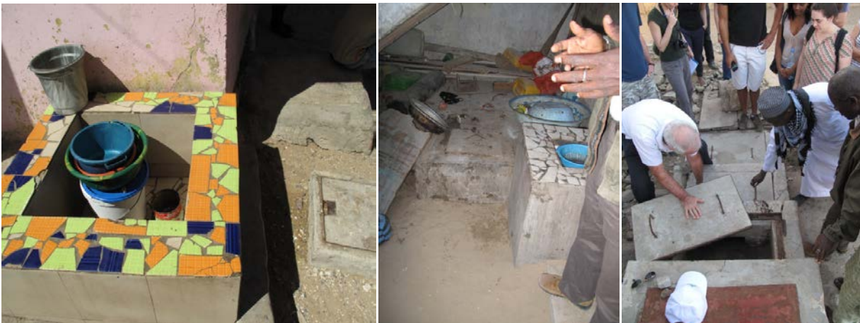
Some of the different solutions used for greywater collection: outside domestic utility sink in Ngor; indoor domestic utility sink with 'sieve' filter in Yoff-Tonghor; communal utility sink in Yoff-Tonghor (not in service)
