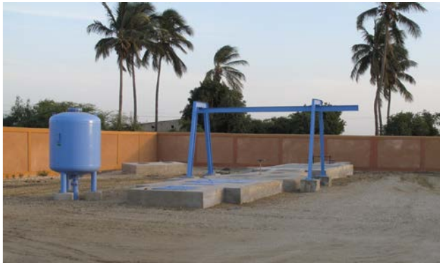
Left: Lift station in Saint-Louis (large capacity as also receives effluent from the conventional sewer system). Right: Emptying a broken down lift station in Ngor using a booster pump.
