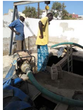
Left: Lift station in Saint-Louis (large capacity as also receives effluent from the conventional sewer system). Right: Emptying a broken down lift station in Ngor using a booster pump.
