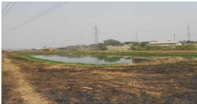
Plate 7: Contractor resources are stretched! - burning of overgrown embankments of anaerobic ponds is resorted to during dry season.
