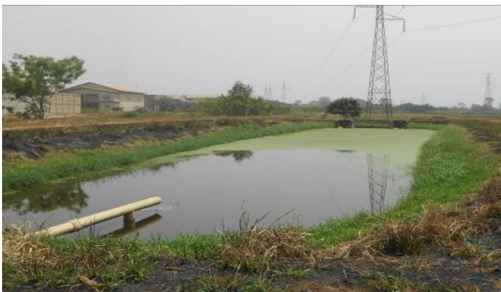
Plate 8: Additional anaerobic pond constructed to cater for institutional connections (Kumasi Polytechnic). Available land around ponds should be preserved against encroachment and for future expansions.
