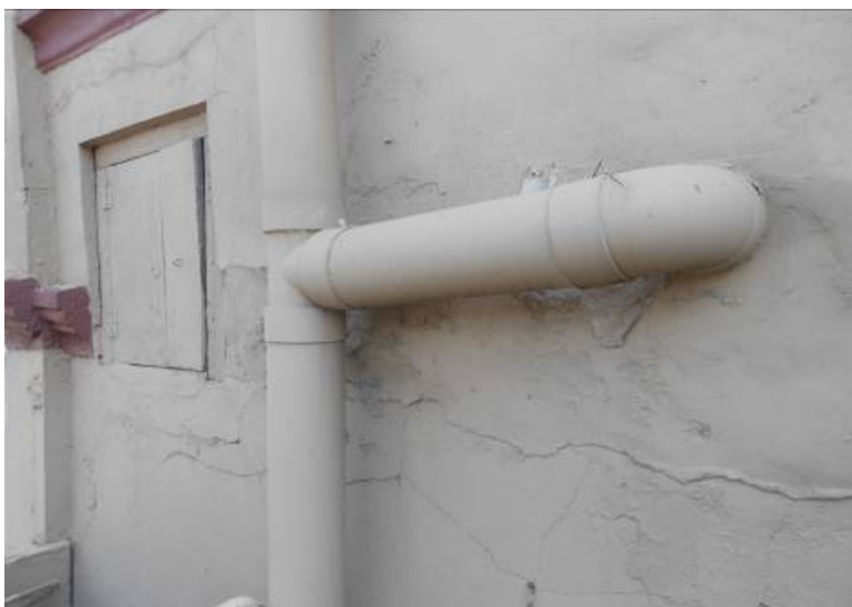
Plate 1: Many houses in Asafo relied on off-site solutions such as pan-latrines. Picture shows old out-of-use nightsoil bucket-chamber and newer sewer connecting a WC.
