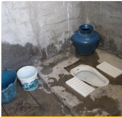
Well-maintained communal toilet in Bangalore
