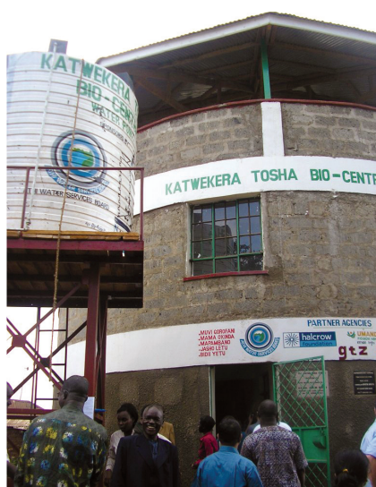
BioCentre facility in Kibera
