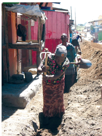
Digging a pipeline trench in Kamere
