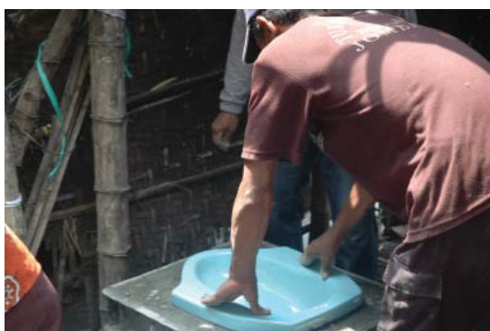
Casting and installing the closet
