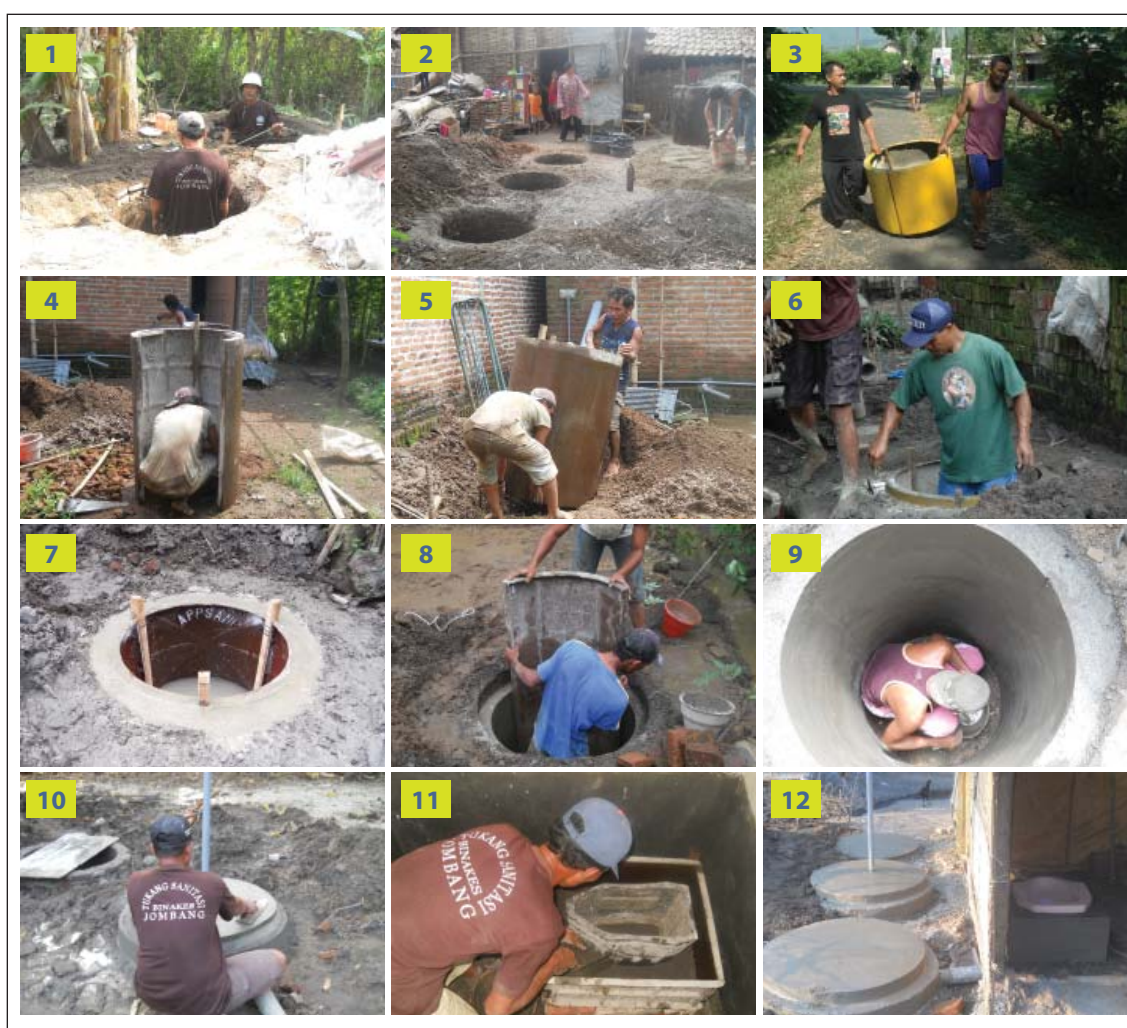
Figure 3.3 Latrine production and installation
