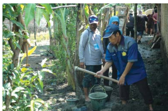
Mixing the sand and cement
