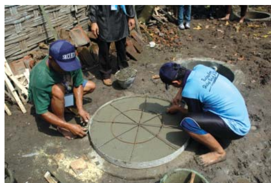
Casting the septic tank lid
