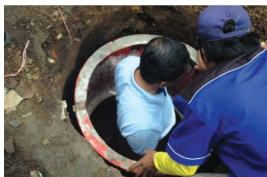
Casting the septic tank
