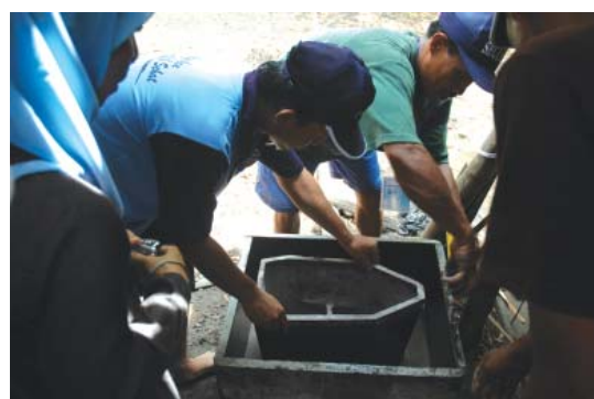
Installing the slab mold
