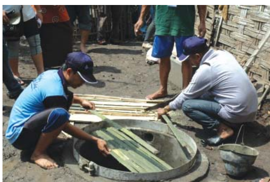
Installing the bamboo framework
