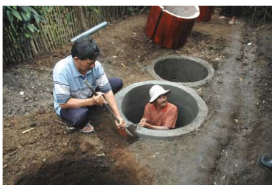
Removing the concrete ring mold
