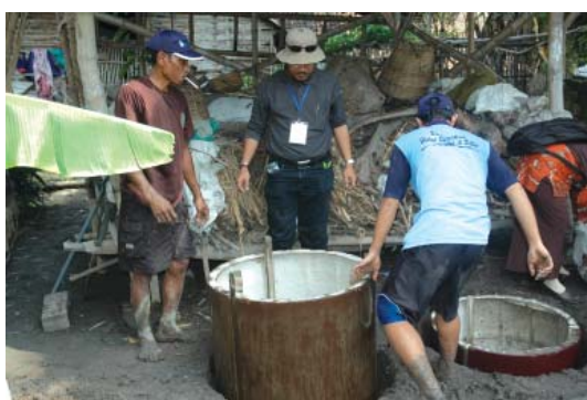
Placing the mold in the hole
