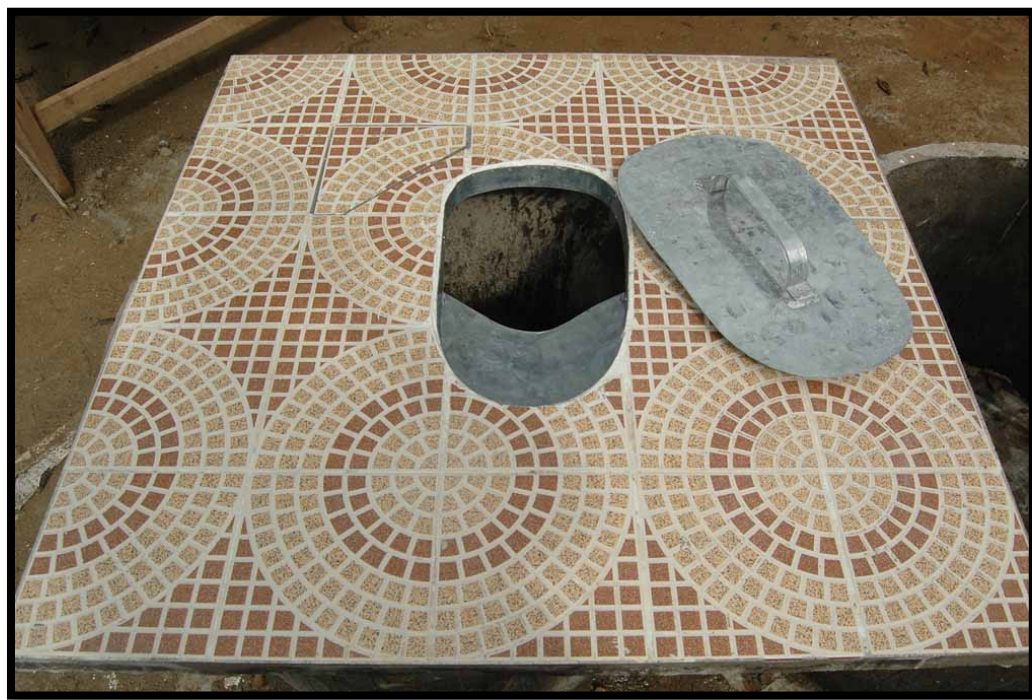
Figure 1: Vit Bor Sai Nam: Upgradable Waterless Toilet (with pit emptying access)
