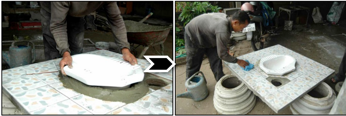
Figure 12 (with alternative pit-access tile construction)
