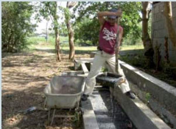
Cleaning the inlet channel. Source: WSP, 2006.
