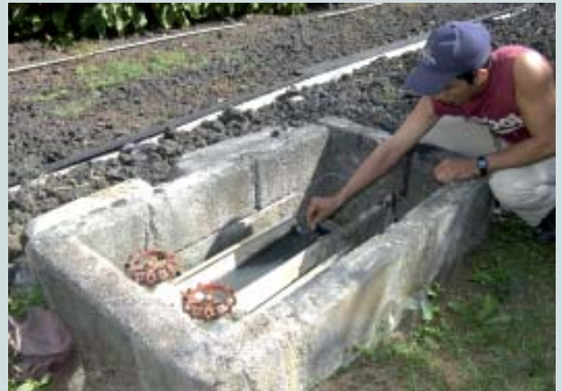
Measuring the flow. Source: WSP, 2006.
