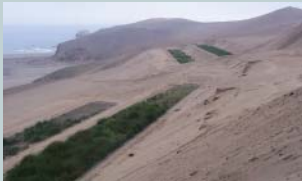
Constructed wetland units at Ventanilla, Lima. Source: Maldonado (2007).
