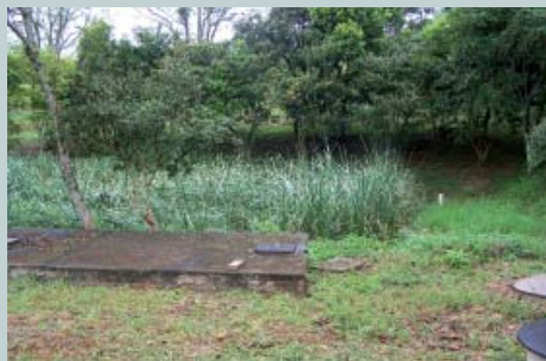
Septic tank and constructed wetland installed at EPAGRI at Florianópolis, Santa Catarina, Brazil. Source: WSP (2007).
