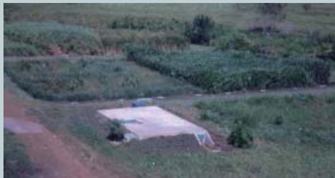
SSHF constructed wetland system at Masaya, Nicaragua. Source: Proyecto Biomasa, 1997.
