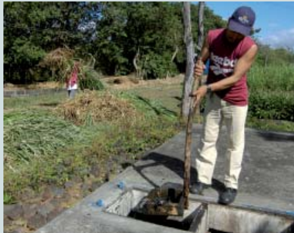
Removing the surface scum from the sedimentation tank. Source: WSP, 2006.
