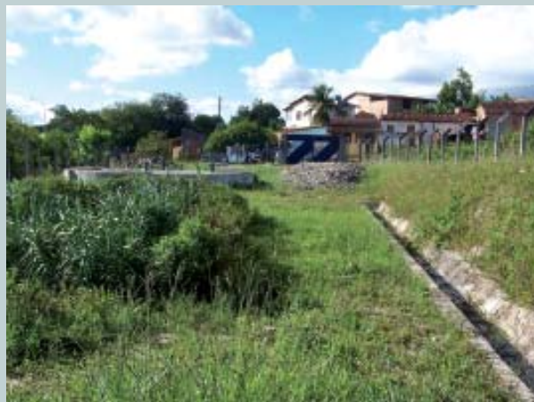
Constructed wetland system at Jardim Petrolar, Alagoinhas, Brazil. Source: WSP (2007).
