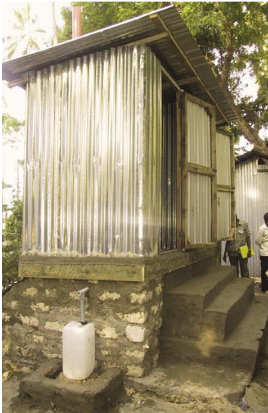
A urine-diversion toilet near Mombasa, Kenya. The urine is collected in the plastic container.
