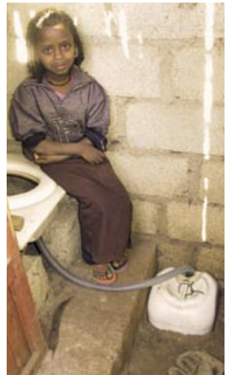
A urine-diversion toilet in Ethiopia.
