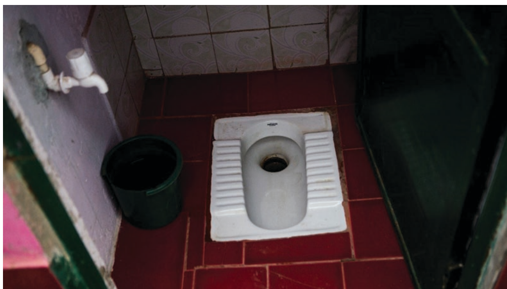
PHOTOGRAPH 16.2. Plastic Latrine Slab over Pit Latrine
