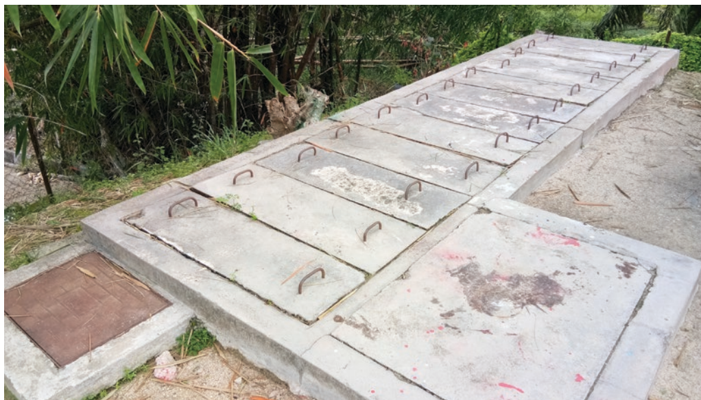
PHOTOGRAPH 17.1. Underground Fecal Sludge Holding Tanks
