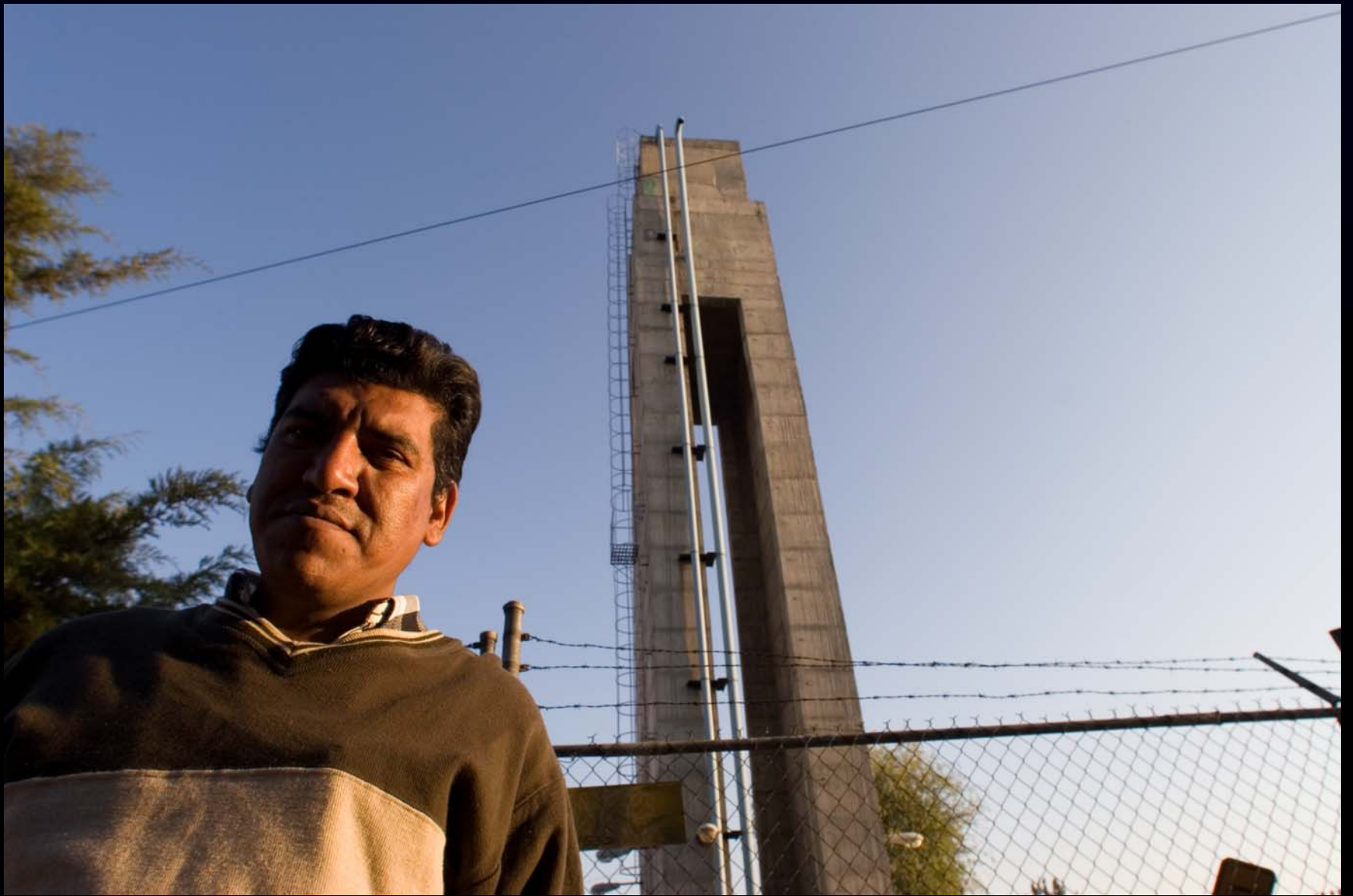
Rogelio Gonzalez manages this pumping and reservoir station that supplies water—for only two hours each day—to the 1,500 residents of the Batallones Rojos apartment complex. ©2006 J. Carl Ganter/Circle of Blue
