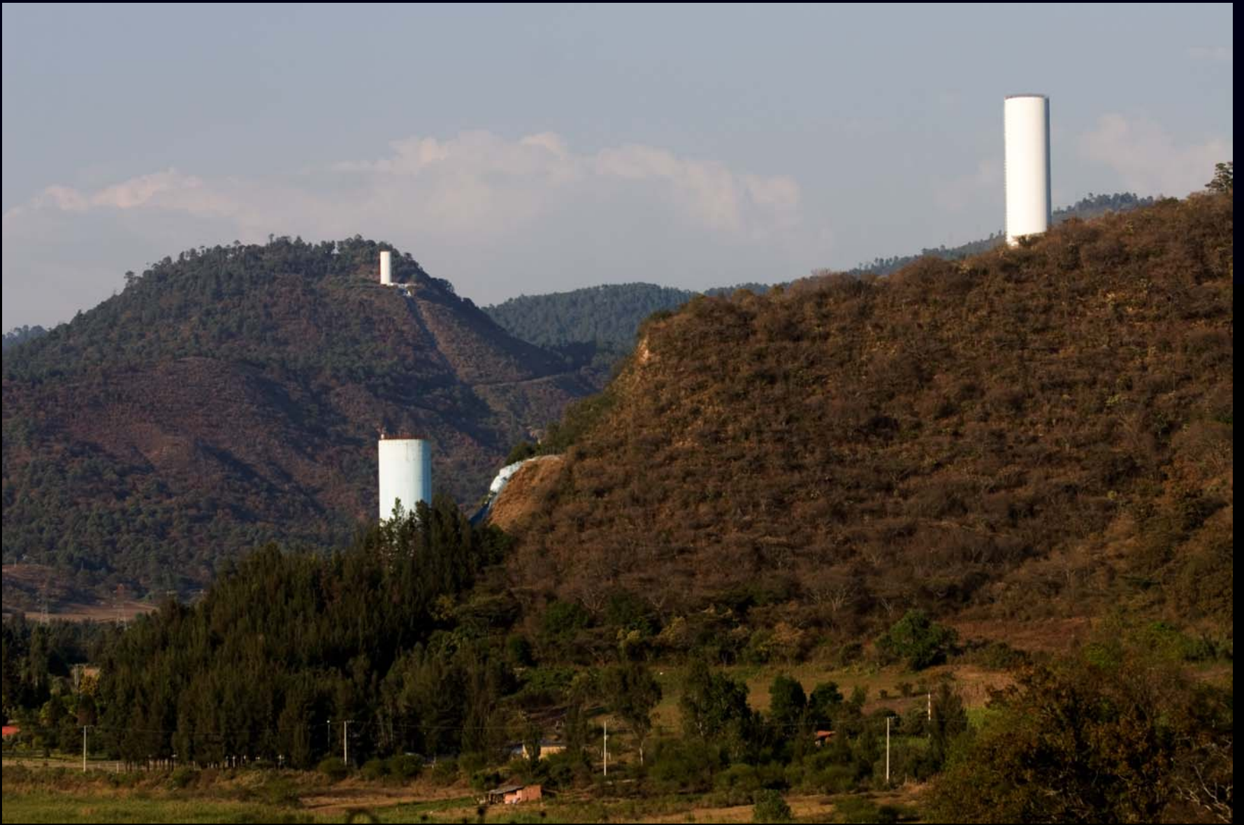
The giant pumping towers of the Cutzamala system force water from Valle de Bravo's man-made Lake Avándaro up and over the mountains toward Mexico City. ©2006 J. Carl Ganter/Circle of Blue
