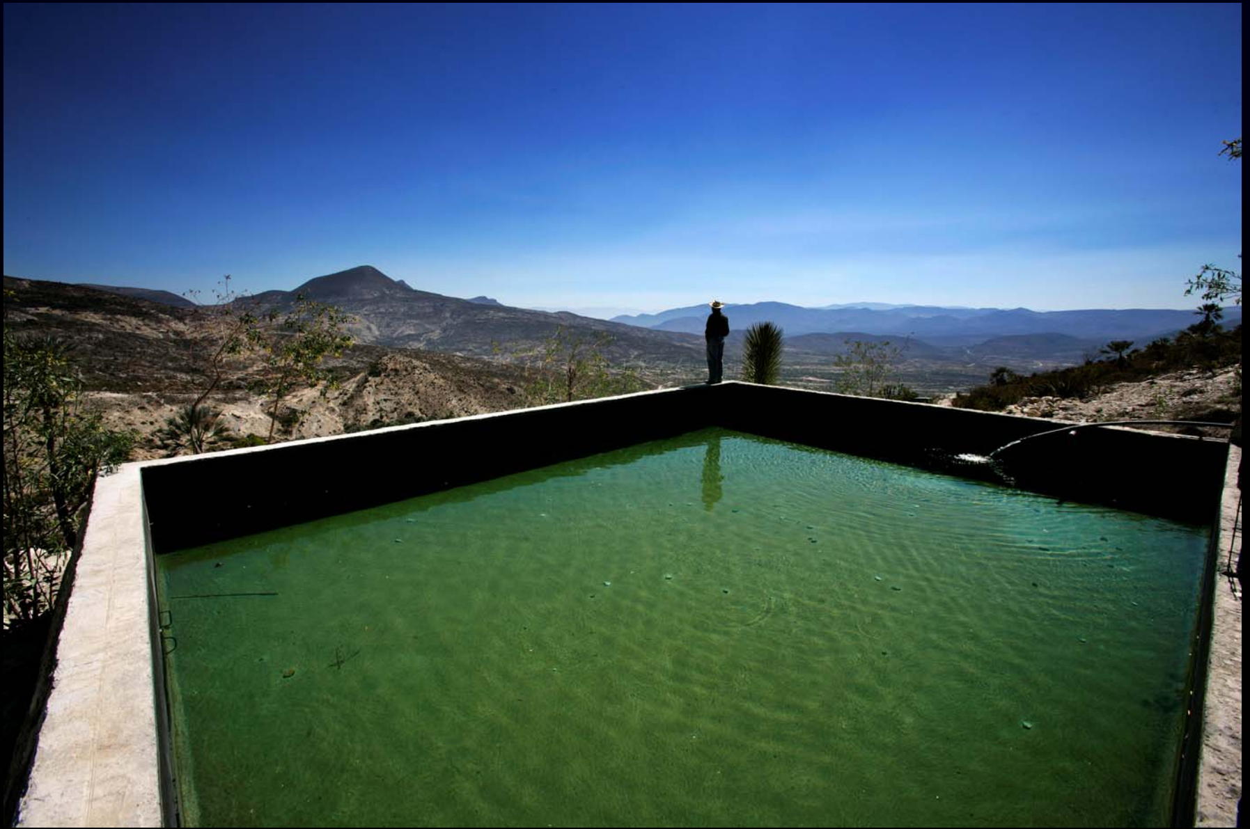
The Carrillo family constructed this water collection reservoir with the help of Alternativas, a regional nonprofit organization. Using a system of pipes and terraces, they are able to deliver precious water to their fields in the valley. ©2006 Brent Stirton/Getty Images for Circle of Blue
