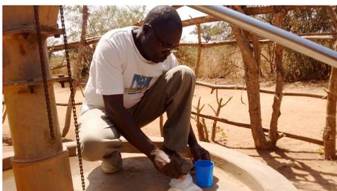
**Photograph 1. HPM calculating chlorine dosage**
