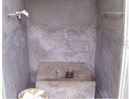
Figure 6. Raised toilet seat with handrails on side walls 6
