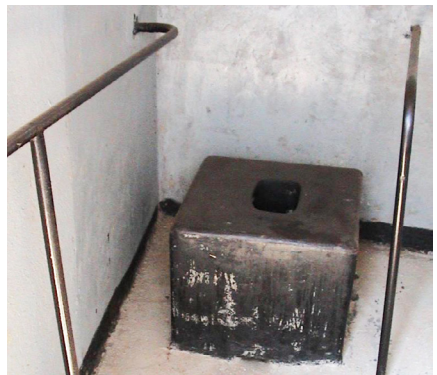
Figure 8. Raised toilet seat with rails fixed to wall and floor 6
