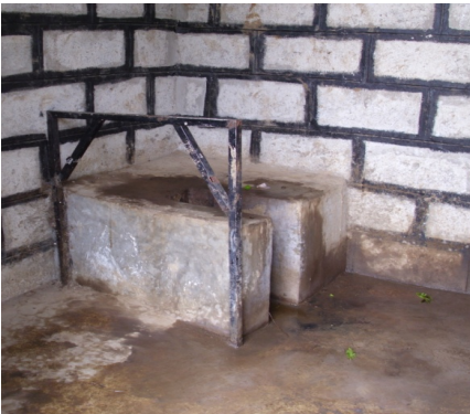
Figure 7. Raised toilet seat with support rail fixed to floor
