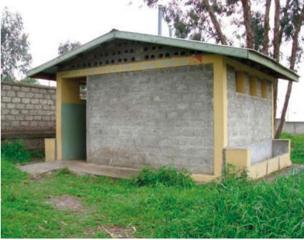
Figure 5. Latrine block with ramp access to entrance on left
