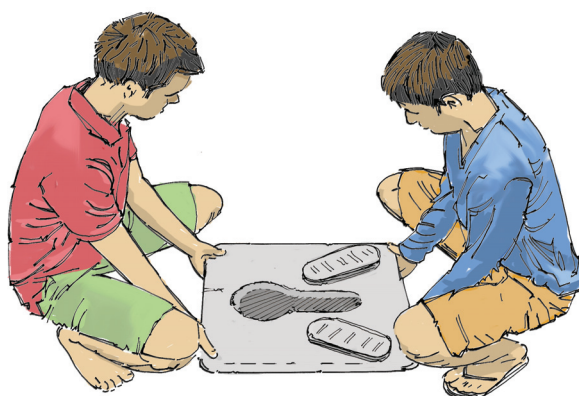
Figure 18. Lifting a sanplat
