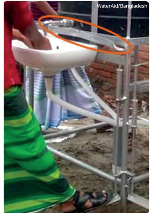
▲ A pedal working in a downward direction, but the lift cock is receiving the upward push by the lever action.
