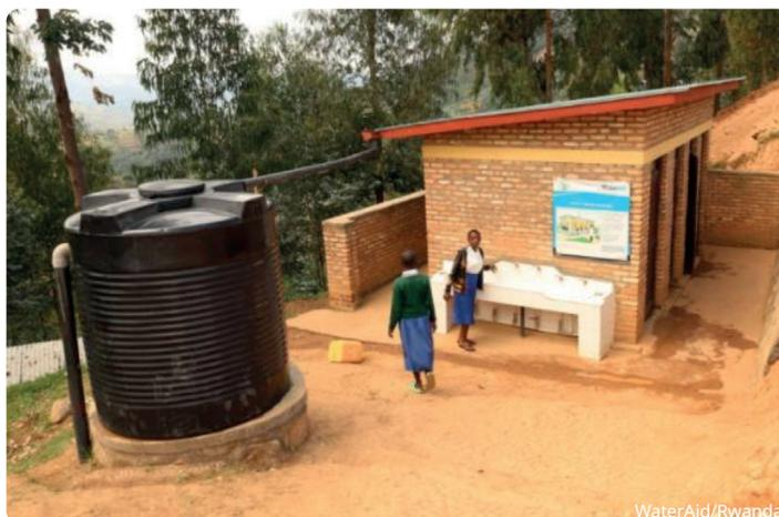
▲ Rainwater harvesting is being used for a handwashing facility for a school in Rusekera.
