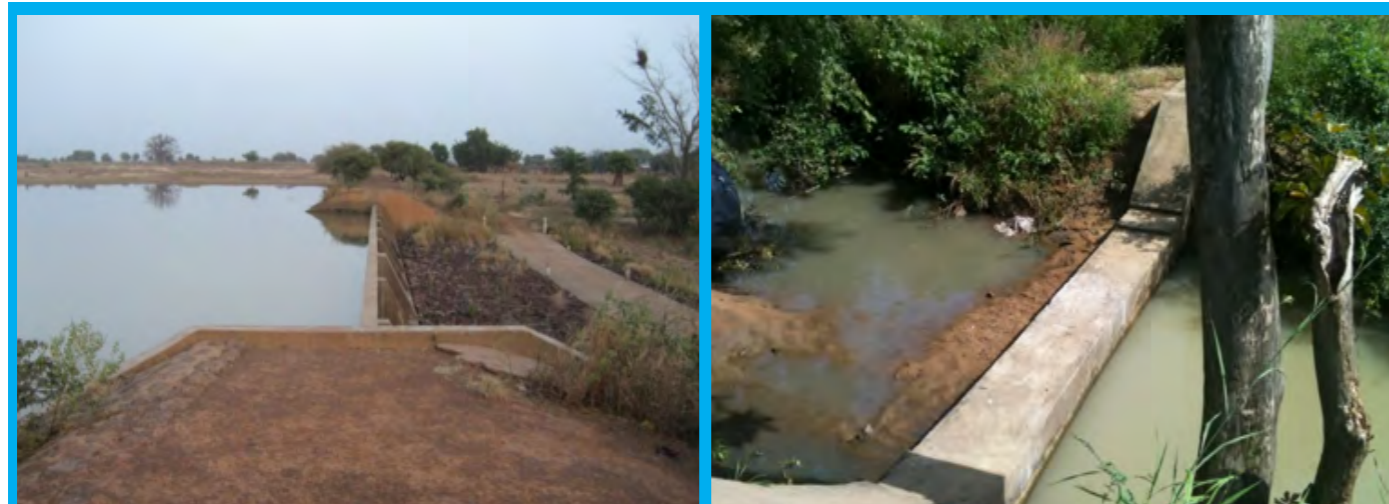
Burkina Faso: small dam and sand dam for groundwater recharge.
