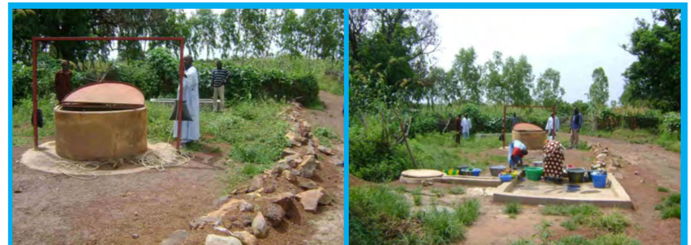
Mali: a large diameter well rehabilitated in Bablebouguou with a washing area for women and troughs for cattle. This well has helped in reducing the pressure on the village borehole for better sustainability.
