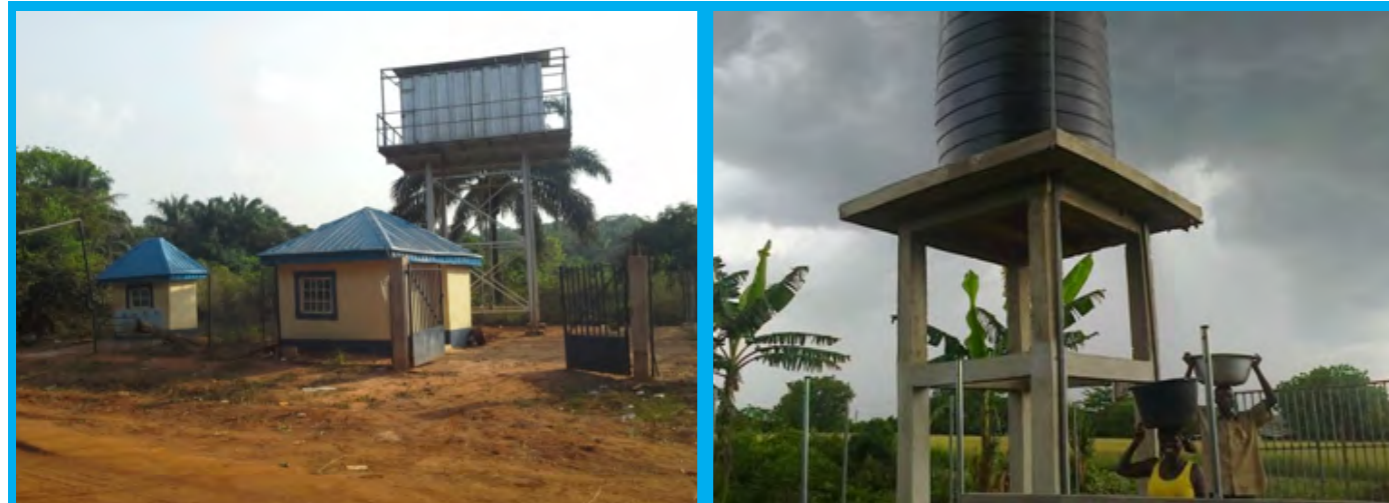
Nigeria (left): view of the Umuofiagu (Enugu State) Solar Water Scheme: Reservoir, Remote control cabin and stand pipe (with elevated standpipe for tanker who collects the water for construction and other needs)
