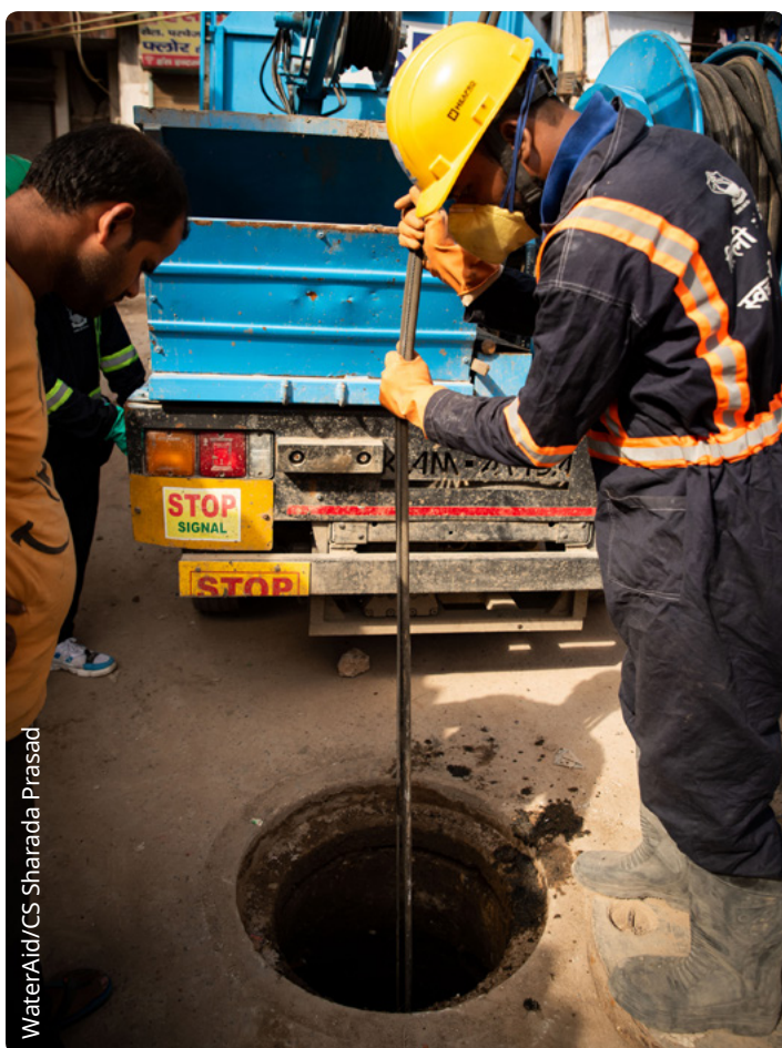
◀ Silt can be removed using a grabbing contraption through mechanised sewer servicing in Delhi, India, 2019.
