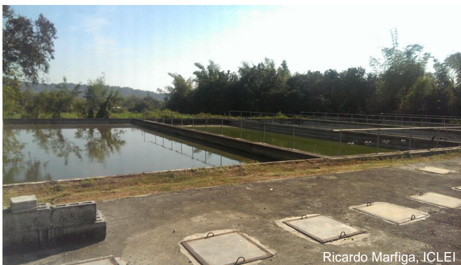
Faecal sludge treatment plant for the whole city.
