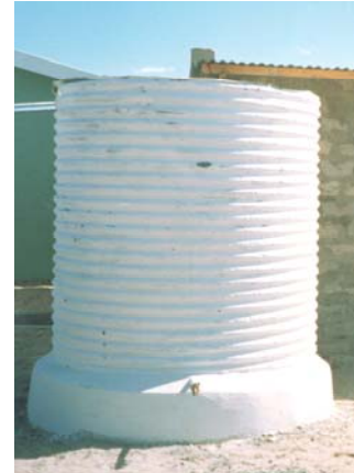
A repaired tank.
