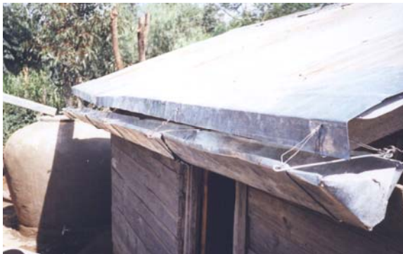
V-shaped gutter suspended from a splash-guard.
