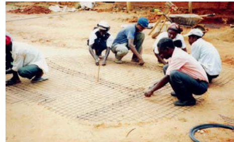
Weld mesh cut to fit
