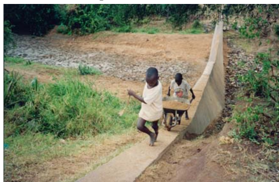
Sand harvesting from a sand dam.
