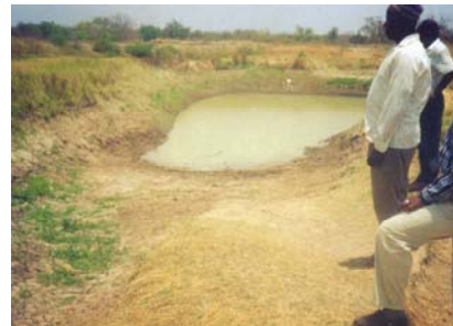
A charco dam in Tanzania.
