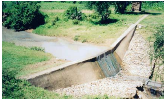
One of the completed sand dams at Kusa.
