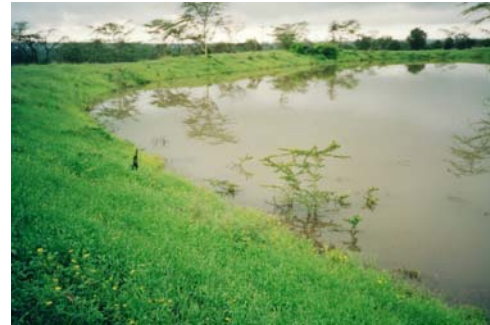
A hillside dam at Lukenya along the Nairobi - Mombasa highway.
