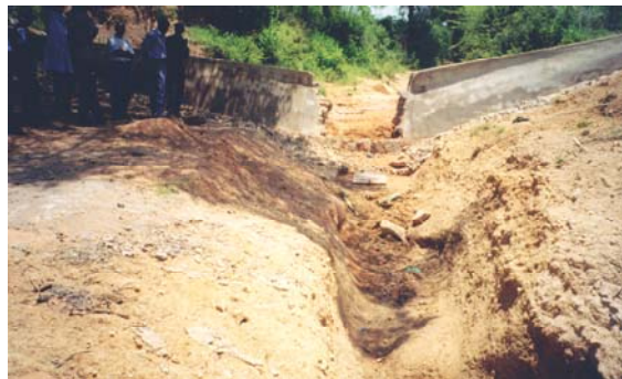
The first stage of a spillway being 30 cm high.
