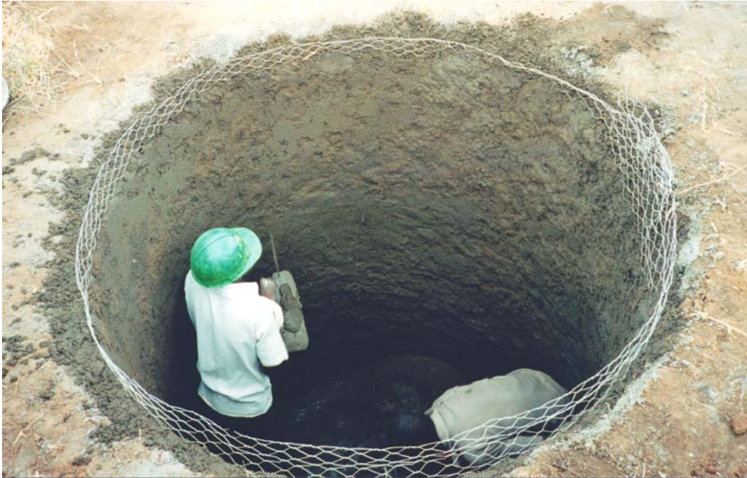
This tank was initially built for storage of ater for construction during a training course at Kibwezi in Kenya in 1997. Upon completion of the training, the tank was equipped with a silt trap and used for harvesting water from a road.
