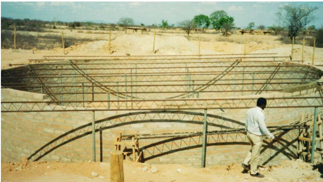
This gigantic cylindrical ground tank was constructed for harvesting rainwater from a large concrete apron near Dodoma in Tanzania in 1992. The tank could also have been used as road catchment of rainwater.
