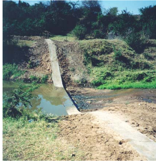
The weir built across the Talek River.
