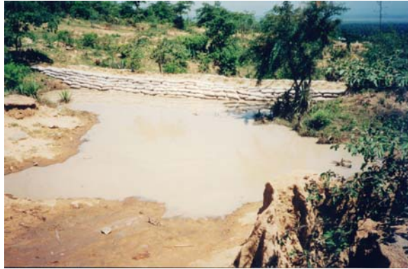
A check dam made of sand bags in a deep gully.
