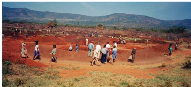
An excavated pan in northern Namibia that harvests run-off water from roads.
