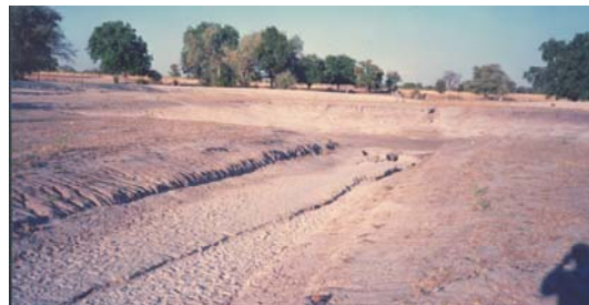
An excavated pan in northern Namibia that harvests run-off water from roads.
