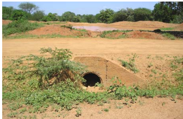
A culvert draining run-off water into a pond.
