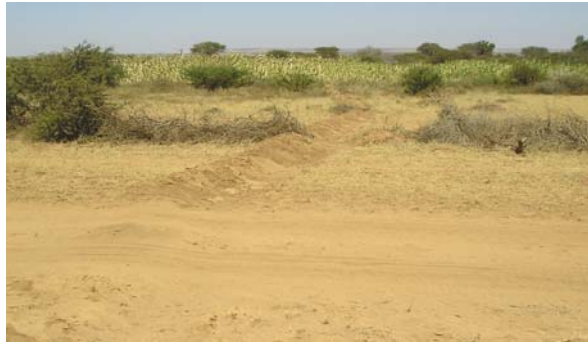
Bump and drain cut manually to irrigate a field.
