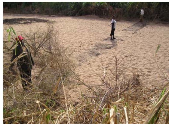
A subsurface dam was built of soil downstream of the Kisasi intake to raise the waterlevel in the sand.
