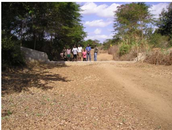
A sand dam with its spillway built in stages downstream of the Mbitini intake to raise and increase the volume of sand and water.
