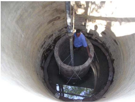
The river-intakes at Kisasi, Mbitini and Ikoo consists of a small diameter hand-dug well sunk inside a wide-diameter hand-dug well.
