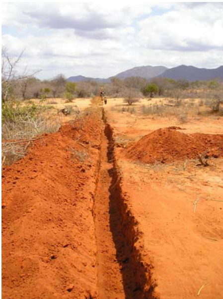
157 km of trenches were excavated and pipes laid in the trenches and back-filled for the 6 water projects.
