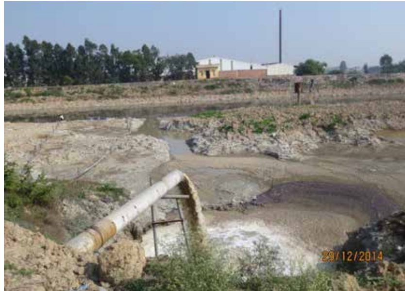
Photo 4: Untreated wastewater discharged into Ngu Huyen Khe River – Bac Ninh, source - CECR
