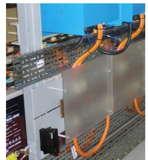
Busbars can be easily made by yourself, you simply need a copper bar where you drill holes in so electrical cables can be connected to the bar. For marine applications use tinned copper busbars. Busbars can be purchased from electrical wholesalers or metal suppliers.
