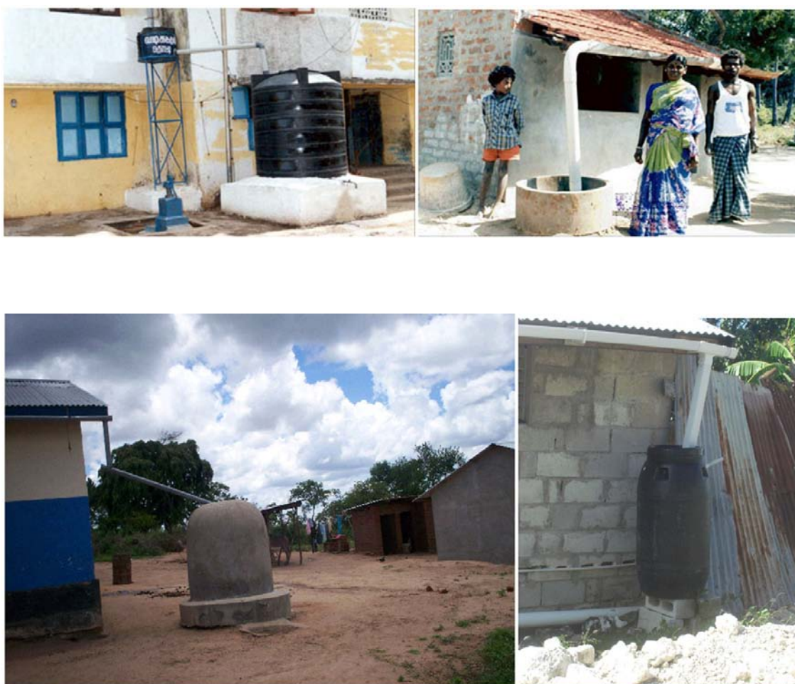
Figure 4.2: Rainwater harvesting from rooftops in Chennai India (12) and Kenya (13) A variety of materials can be used to store the collected water. Plastic vessels are often available in the local market and are light to transport and generally fairly cheap. Where these are not available, in-situ construction using light-weight ferro-cement is a good alternative. Underground tanks may be preferred in some locations due to greater storage capacity and the fact that water supplies tend to remain cooler.
