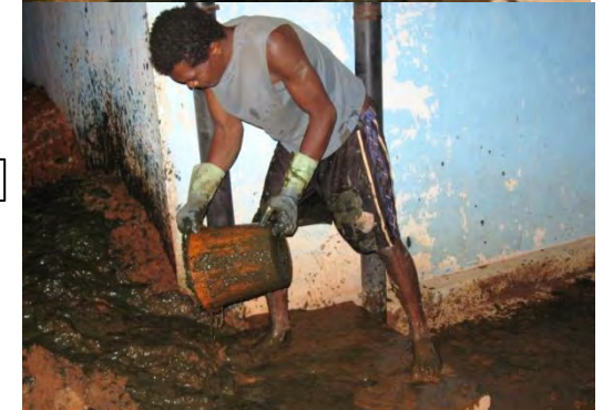
Removing the sludge
