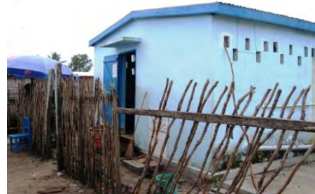
The toilet and shower unit
