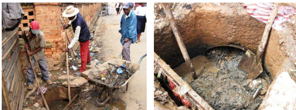
Dredging of drainage canals and sewers by the municipality’s mobile teams (Ambositra)
