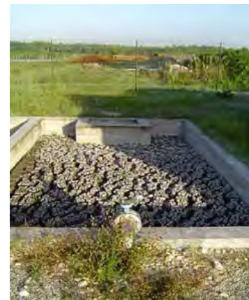
View of a drying bed
