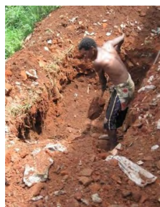
Digging a trench for burying the sludge behind the toilet and shower unit in Alakamisy.
