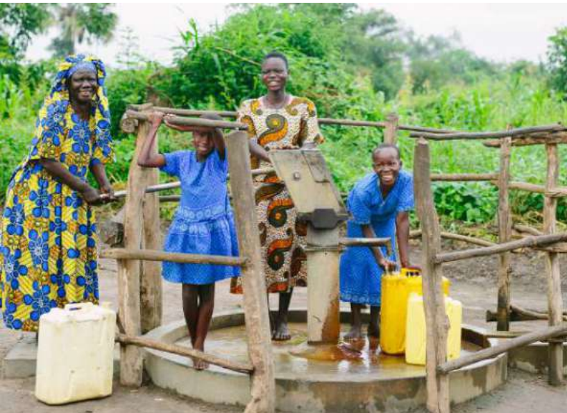
Figure 18. Handpump equipped with an integrated remote sensor (in black casing) developed by charity: water (Source: Hazel & Pine and Esther Havens)
