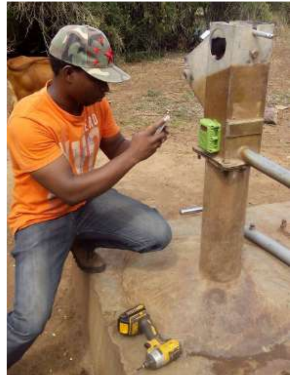
Figure 17. A satellite-enabled Virridy remote handpump sensor, mounted in green casing (Source:Virridy)
