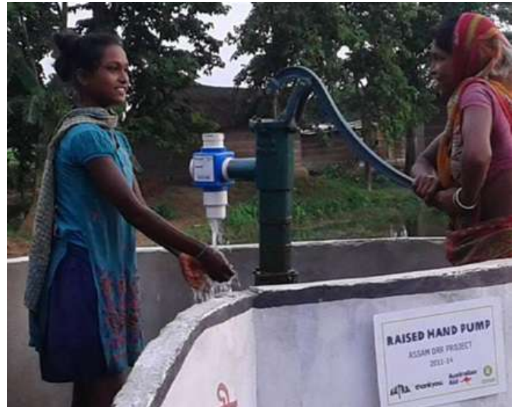
Figure 8. PurAll Handpump chlorinator (Source: EaSol Private Limited)
