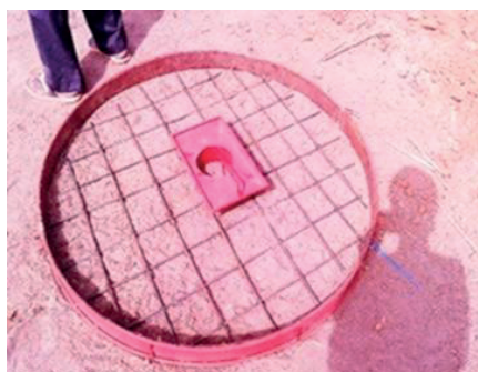
Ferraillage dalle normale
