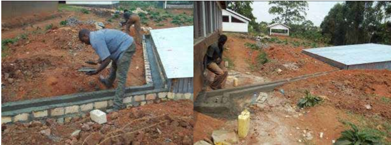
Figure 11: Drainage channels under construction (left) and with collection box completed (right)
