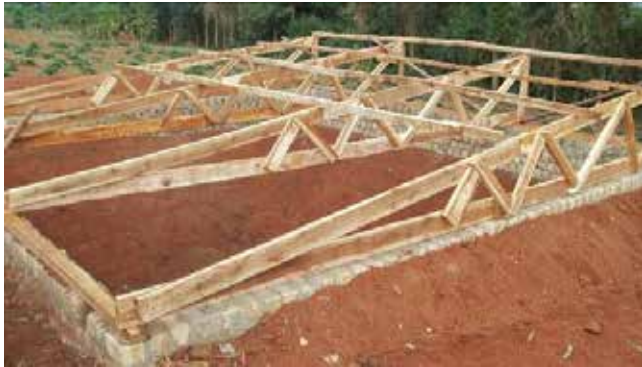
Figure 8: Erecting timber frames on the plinth wall for pond covering
