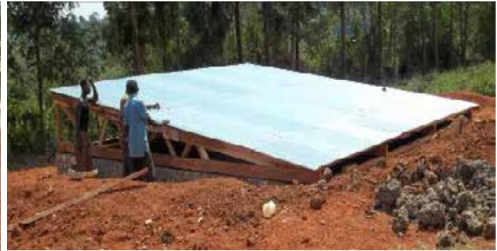
Figure 9: Fixing roofing sheet covering over the pond
