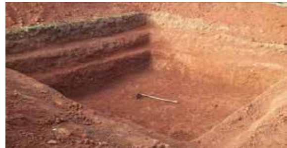
Figure 4: Stepped excavation for pond
