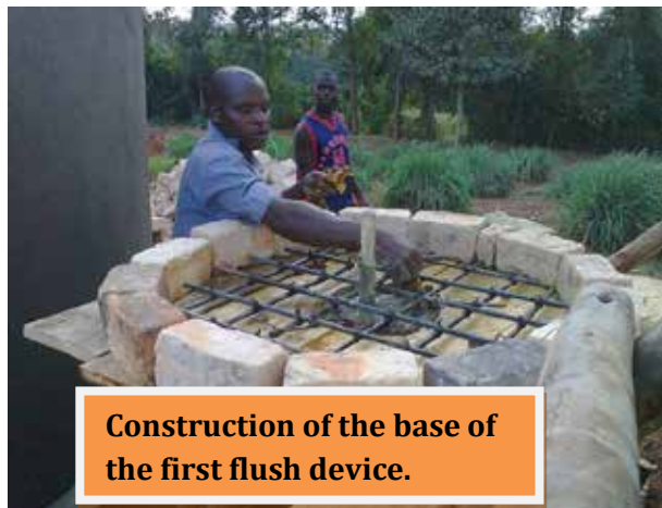
Setting of the first flush device base
