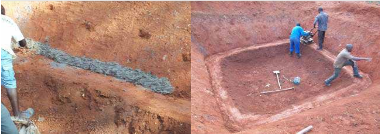
Figure 6: Apply a layer of puddle clay (left) then apply a layer of cement/Murram and compact (right)
