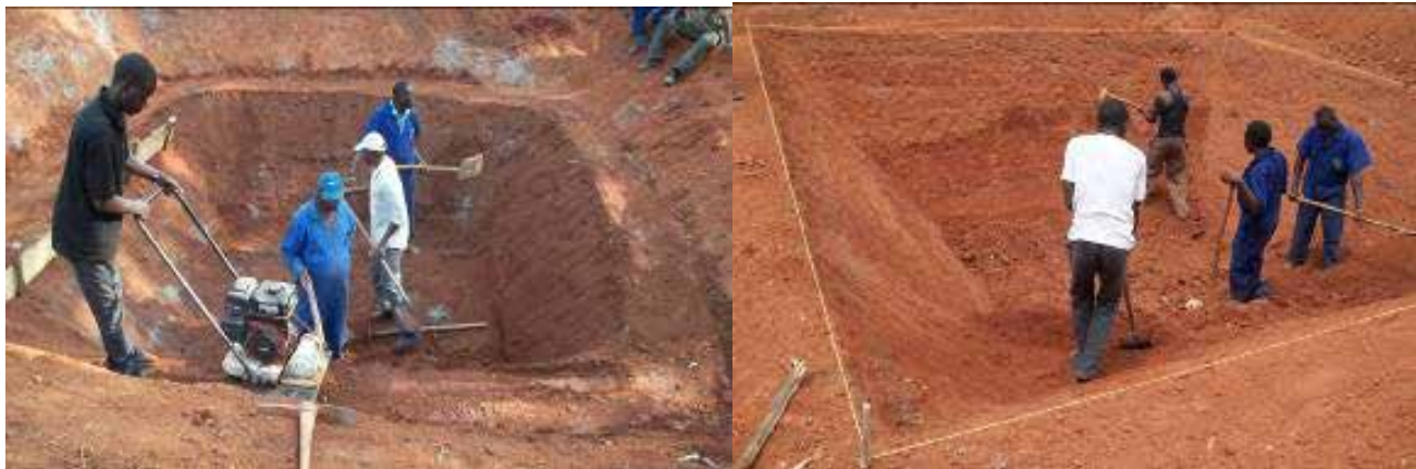
Figure 7: Continue compaction in layers up to the top (left) and trim off excess compacted Murram (right)
