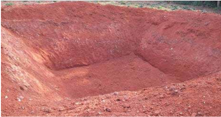
Figure 5: Excavation completed by cutting off the steps from the sides of the pond
