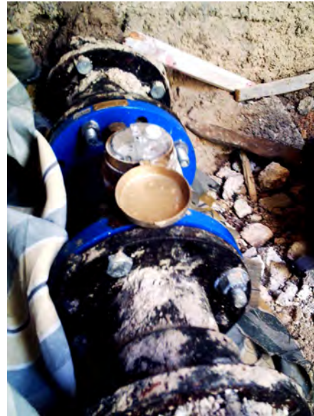
Pilot Area Muhandesien Subdivision, Bulk Water Meter 100mm Inlet
