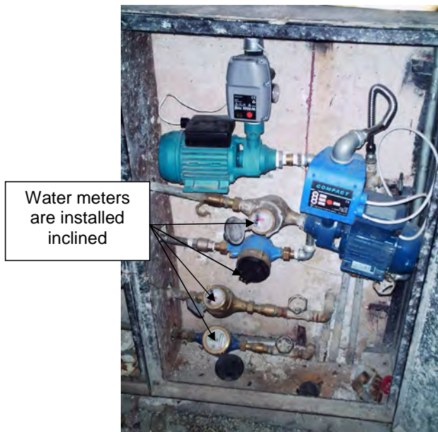
Pilot Area Muhandesien Subdivision, Typical Water Meter Tree
