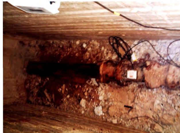
Pilot Area Muhandesien Subdivision, Bulk Water Meter 150mm Inlet
