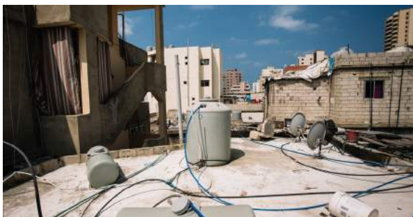
Private tanks in Mar Elias camp. ©2017 UNRWA
