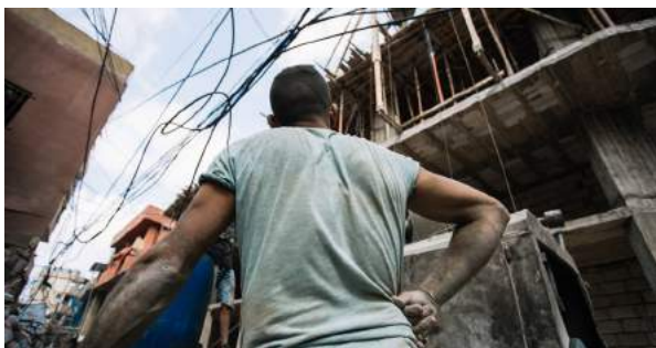
Construction site and infrastructure workers. ©2017 UNRWA
