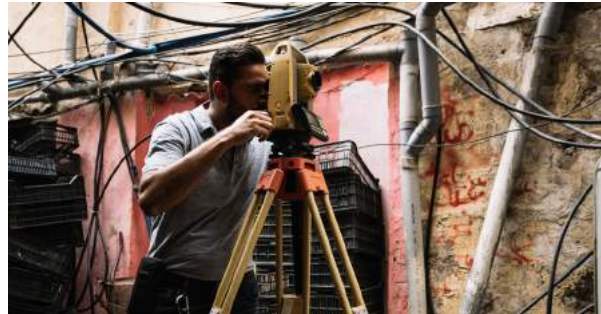
Surveying engineering work. ©2017 UNRWA
