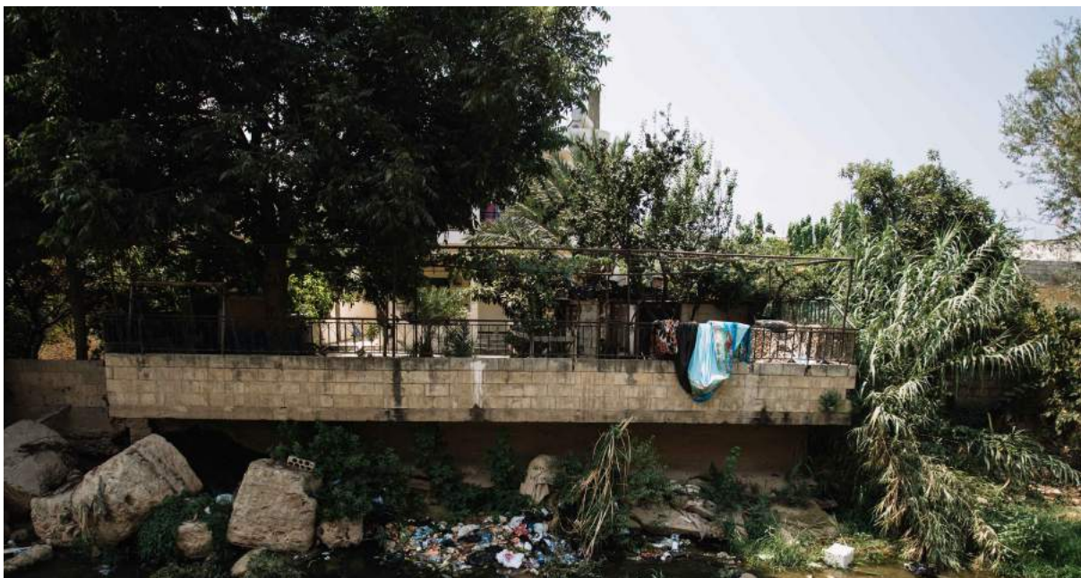
Drainage problems after heavy rains. ©2017 UNRWA
