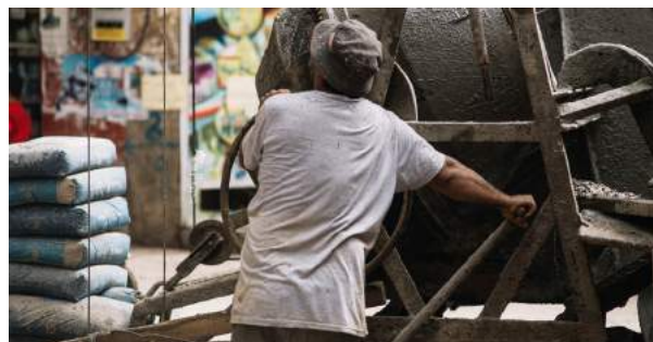
Construction site and infrastructure workers. ©2017 UNRWA
