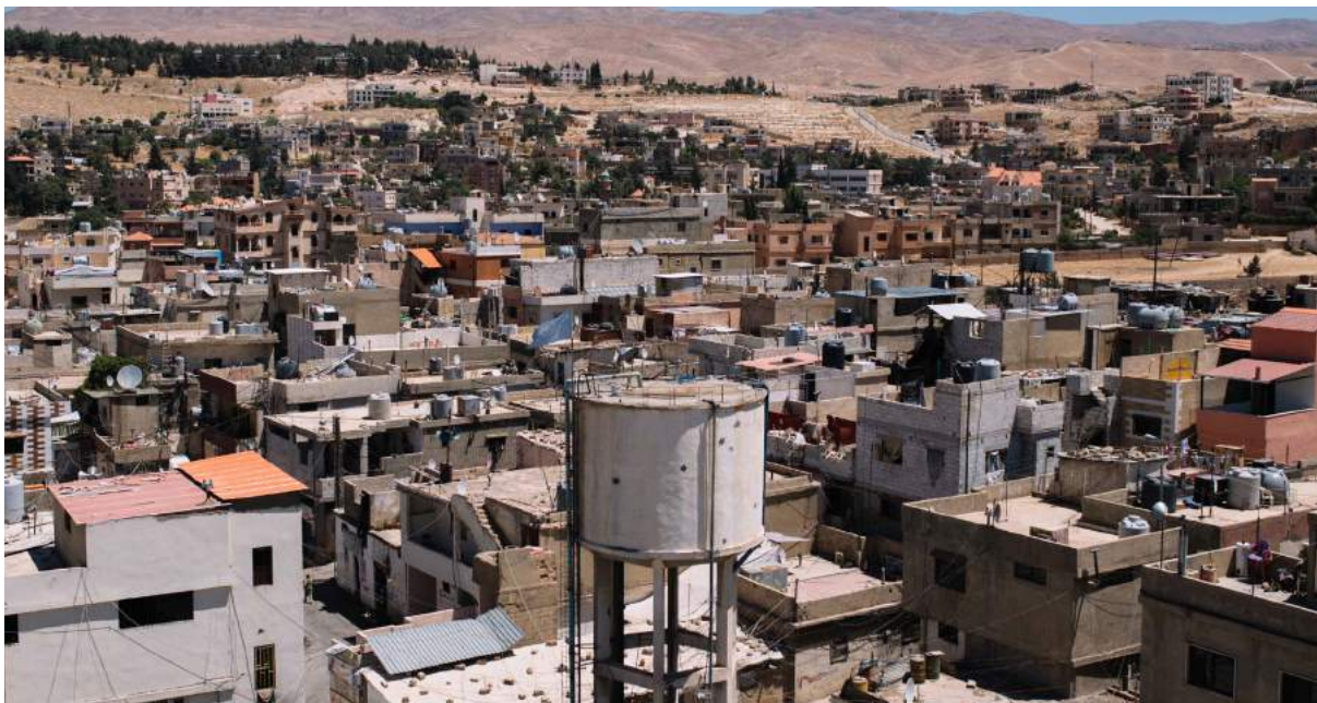
Water tank in Wavel camp. ©2017 UNRWA
