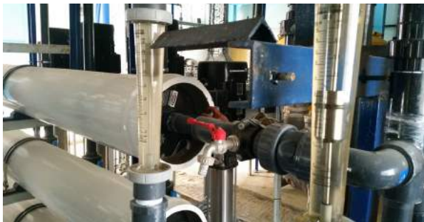
Reverse osmosis in Shatila camp. ©2017 UNRWA
