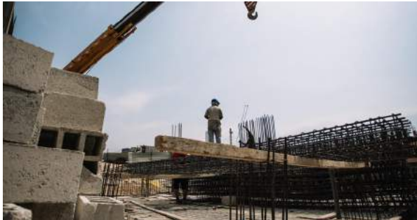
Nahr El Bared reconstruction project. ©2017 UNRWA
