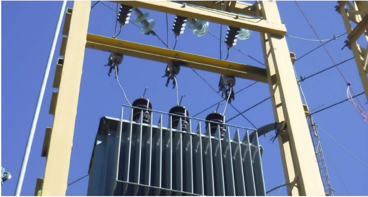
Electrical Transformer in Wavel. ©2017 UNRWA
