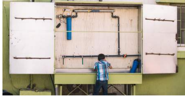
Reverse Osmosis distribution tap in Shatila. ©2017 UNRWA
