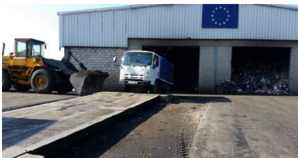
Ain Baal Solid Waste plant in Tyre area. ©2017 UNRWA
