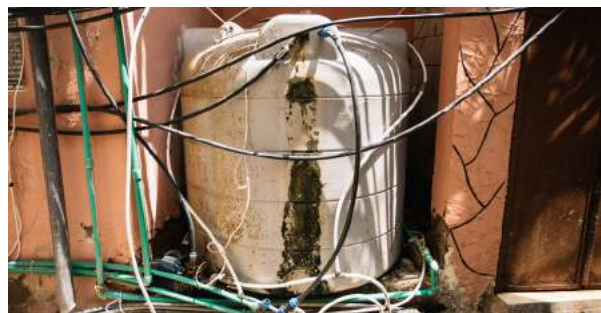
Individual water tank and booster pump. ©2017 UNRWA
