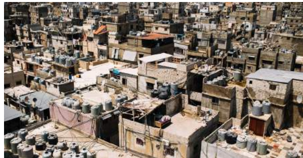
Roofs in Shatila camp. ©2017 UNRWA
