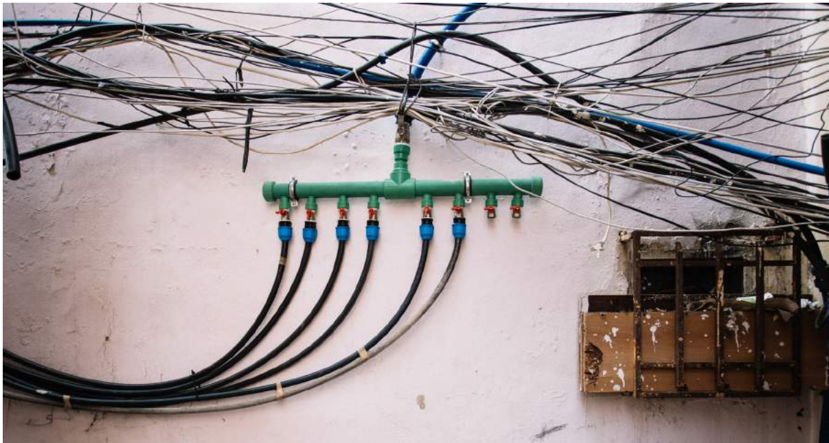
Water connections in Burj Barajneh camp. ©2017 UNRWA
