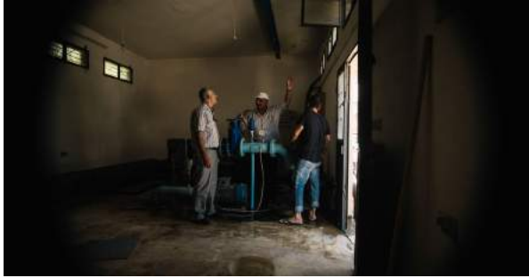
Water borehole inspection. ©2017 UNRWA
