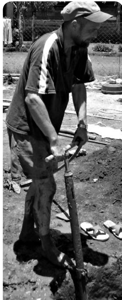
Fig. 2.33 Hand-operated mud pump
