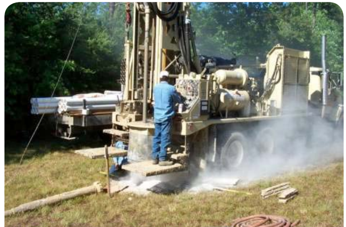
Fig. 2.11 Down-the-hole hammer drilling
