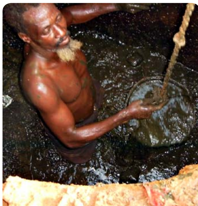
Fig. 5.1 Manual pit emptying
