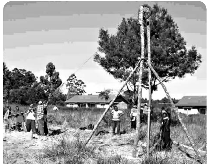
Fig. 2.19 Stonehammer drilling in action
