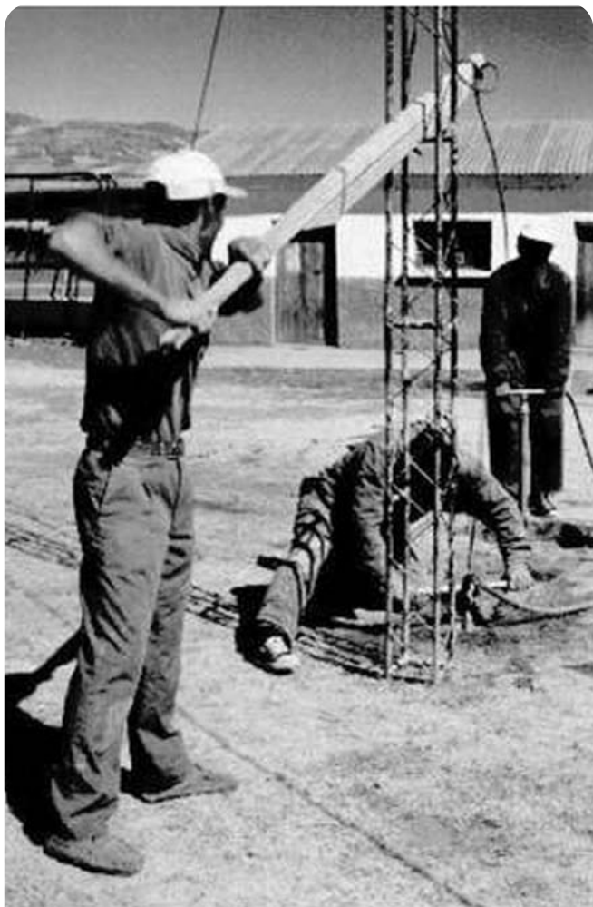
Fig. 2.31 EMAS drilling
