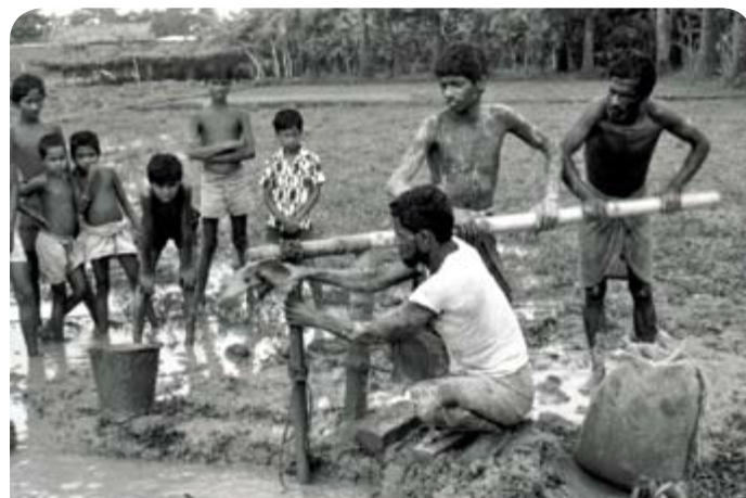
Fig. 2.23 Sludging in West Bengal
