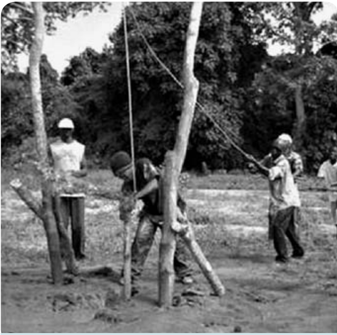
Fig. 2.24 Reaming of a Baptist drilled hole by sludging
