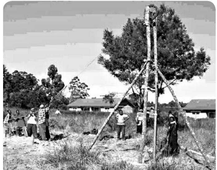
Fig. 2.19 Stonehammer drilling in action
