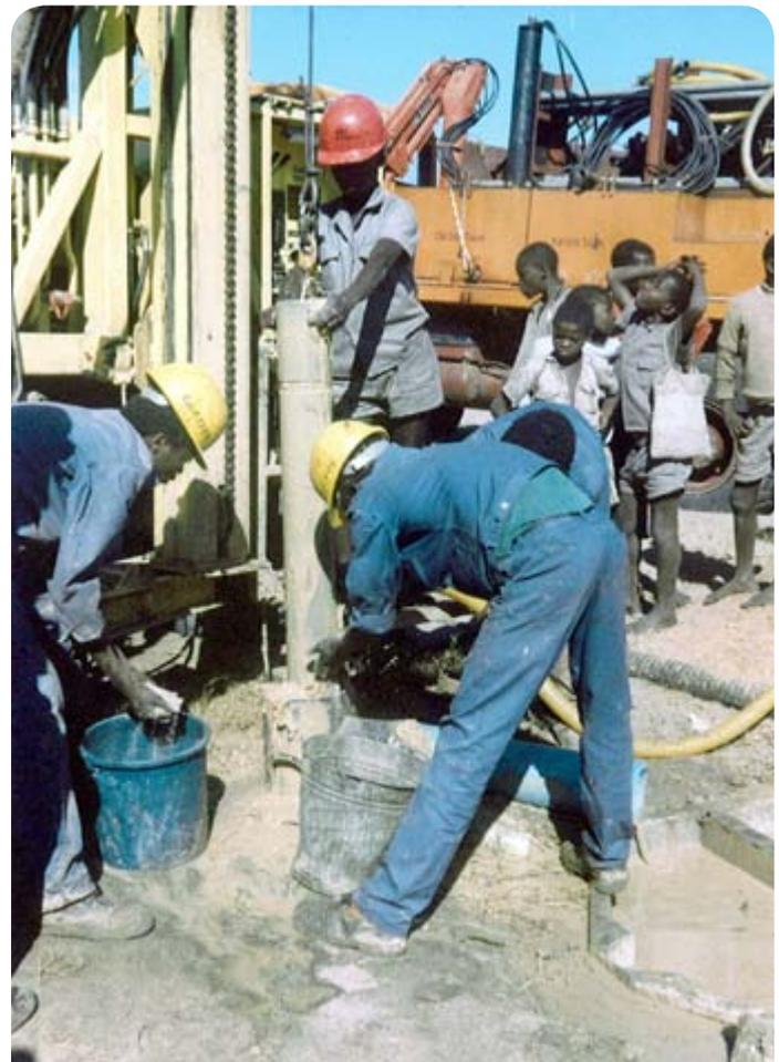
Fig. 2.43 Placing the gravel pack, Zambia © S. Sutton
