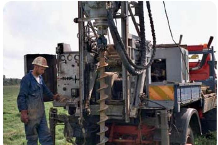
Fig. 2.6 Auger drilling
