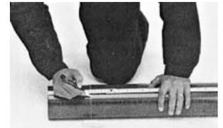
If one of the pipes needs to be cut to fit, mark the exact position (a line around the whole pipe) and cut along the line with a hacksaw. Remove the burrs with a knife.
