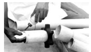
Note that the bell-ends of standard pipes are slightly tapered and designed so that the pipe cannot be inserted dry into the bell-end. Insertion is only possible once the cement has been applied. This property is used to check for correct dimensional
