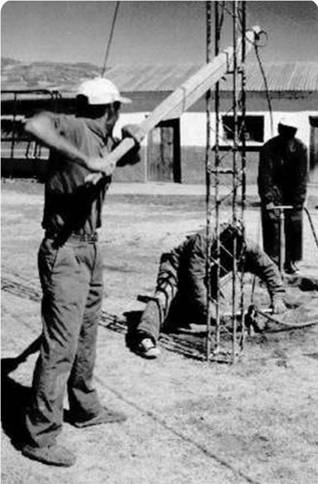
Fig. 2.31 EMAS drilling
