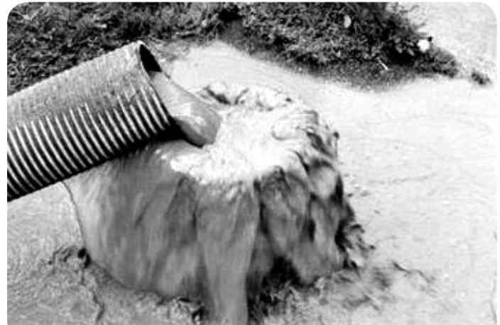
Fig. 2.45 Water pumped before development
