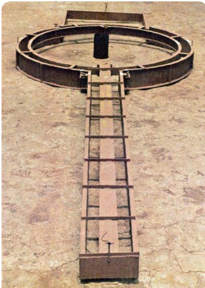
Fig. 2.53 Mould for the platform, Tanzania © UNICEF
