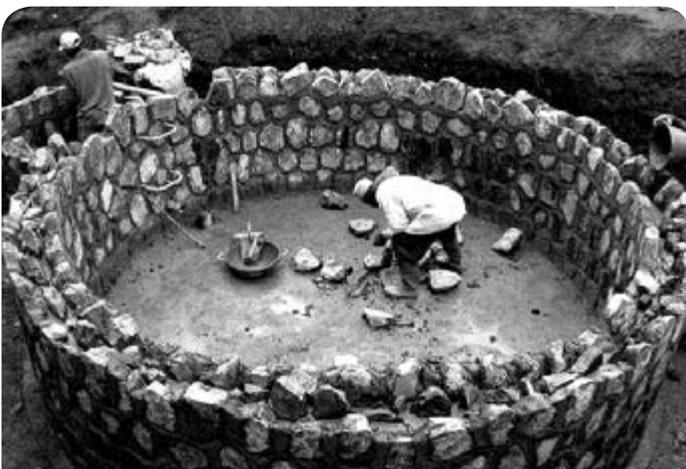
Fig. 4.27 Masonry groundwater tank, Lesotho
