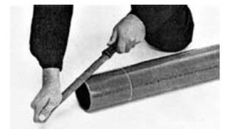
All pipe ends (outside) up to the marked line and all bell-ends (inside) should be slightly roughened with sandpaper until the surface loses its sheen (until it has a matte appearance).
