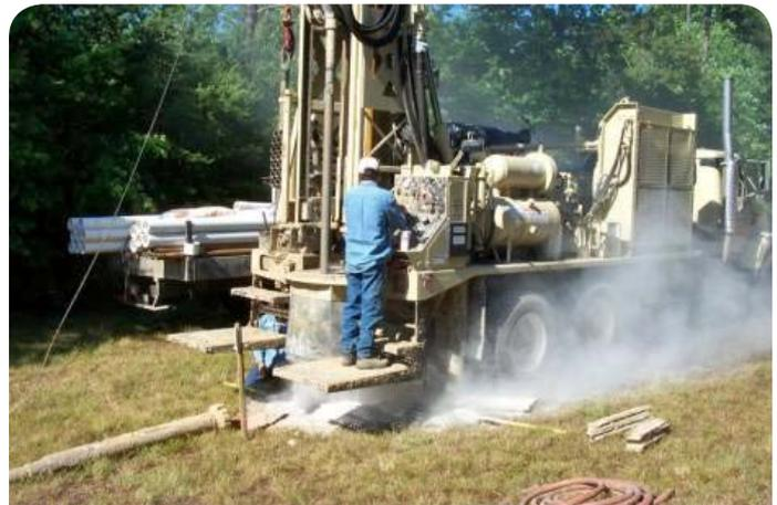
Fig. 2.11 Down-the-hole hammer drilling
