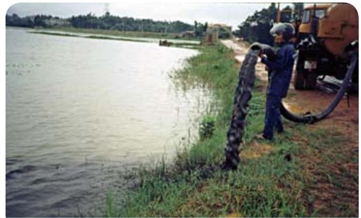
Fig. 5.11 Sludge discharge in a pond, Vietnam © Sandec
