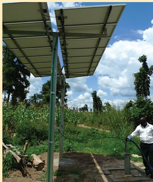
UNICEF-supported solar powered water system in Uganda. © UNICEF Uganda/2015
