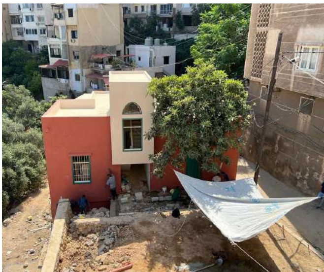
Building nearly completed rehabilitation, Beirut, Lebanon - UN Habitat, 2022
