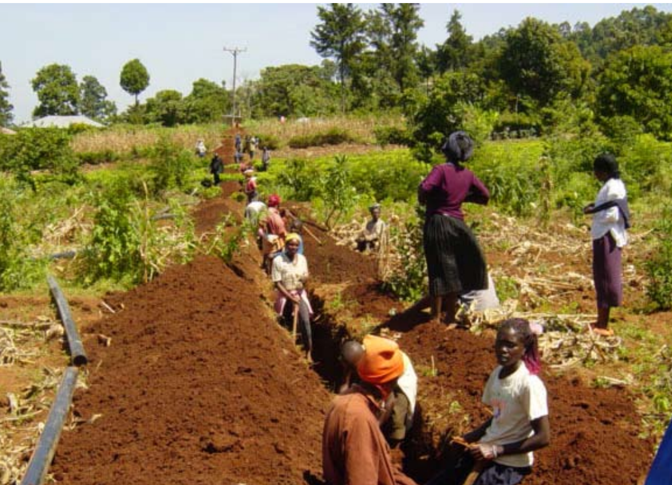
Community joint effort in digging trenches for water pipes. Photo © UN-Habitat
