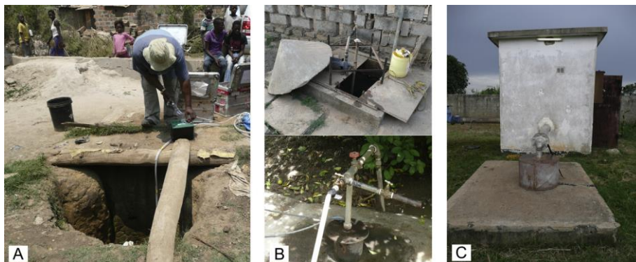
Figure 3-14: Relating groundwater source vulnerability to land use: (A) a vulnerable, unlined, shallow well adjacent to the road in a lower cost housing area; (B) a shallow well and a borehole with protective headworks, located in gated properties within higher cost areas; (C) a fully-sealed public water supply borehole within a secure compound in the peri-urban Mukobeko wellfield in Zambia (Sorensen et al., 2015a).
