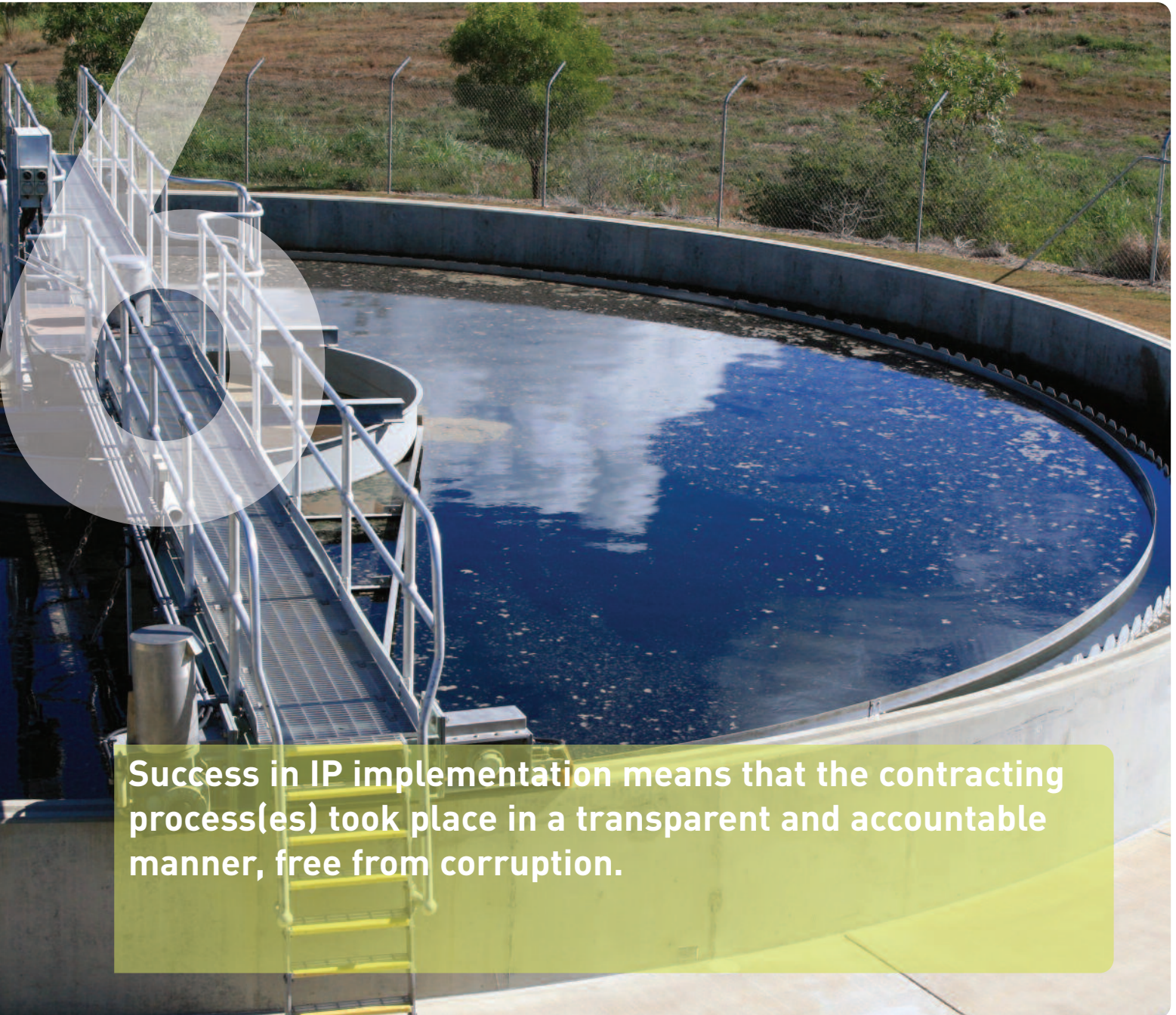
Clarifier tank at a Sewage Treatment Plant. © pampix/istock
