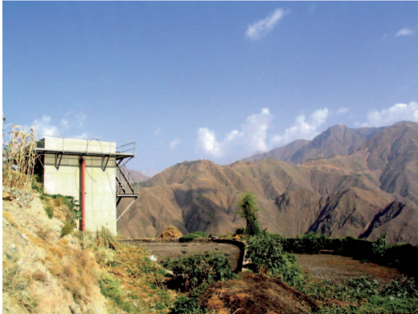
Figure 6.2 Imhoff Tank and sludge drying beds at Hajjah
