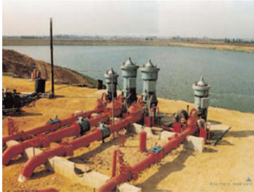
Figure 21.4 Groundwater recharge of reclaimed water for treatment, storage and agricultural irrigation in Israel
