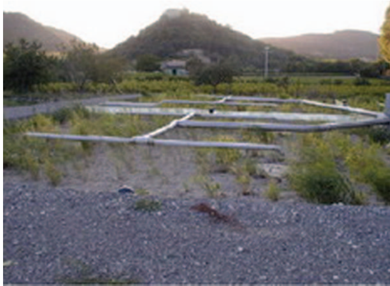
Figure 14.3 The first stage unit from the Phragmifiltre® of Saint Thomé (SINT, 2004)
