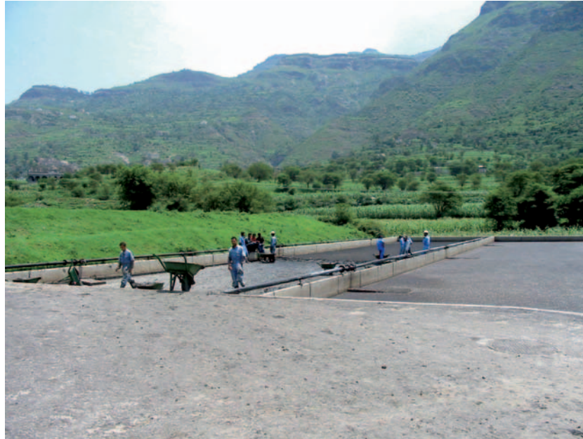
Figure 6.4 Manual lifting of sludge from drying beds at Ibb wastewater treatment plant
