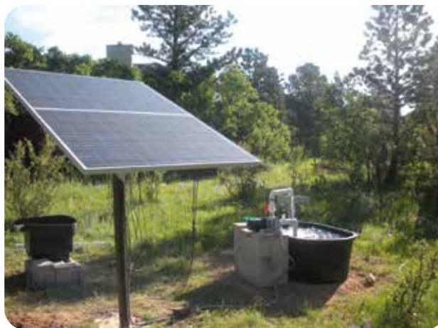
Submersible Water Pump System
