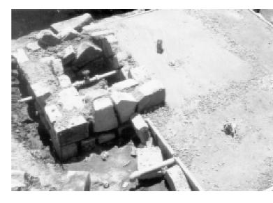
Building the wall according to the required bonding.
