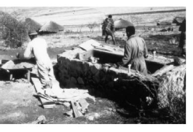
5. During the time of plastering the pointing of the outside wall can be done.
