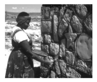
Pointing can be carried out as the construction of the blockwork proceeds, using ordinary mortar in which the blocks are bedded. This type of pointing is called struck jointing and is much cheaper than the pointing methods described below. Another method is to finish the masonry work first and then to make the pointing work with a 1:2 cement mortar later. The joints must be racked out to a depth of about 1 to 1.5 cm, brushed, washed and filled with a 1 part cement and 2 part sand mortar.
