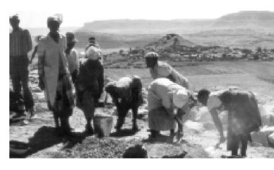
Hand mixing does not require much equipment, but a lot of man power. A batch to be hand mixed should not be larger than about 0.5 m<sup>3</sup>. Concrete should never be mixed on soil because of the proved danger of contamination by organic matters. A levelled platform has to be prepared to prevent water or fluid material from flowing out of the mixture.
