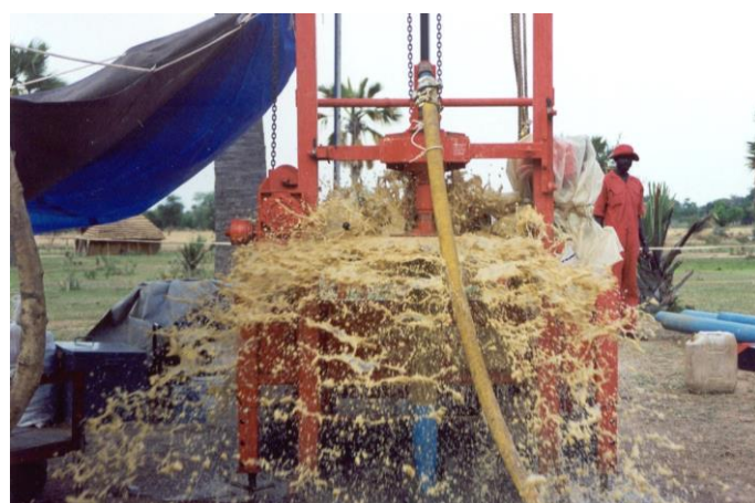
Figure 5: Well Development using Compressed Air
