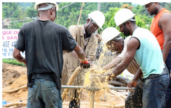
Figure 14 Rota-jetting equipment used in the DRC (Source: UNICEF)
