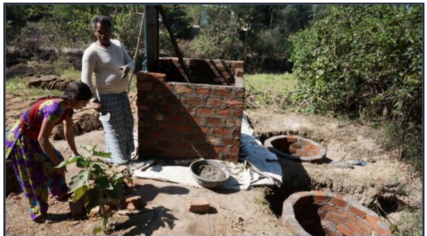
An Indian government latrine under construction
