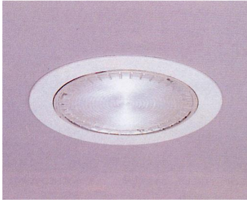
Illustration 7: Non-suspended PLC downlight, mounted onto ceiling
