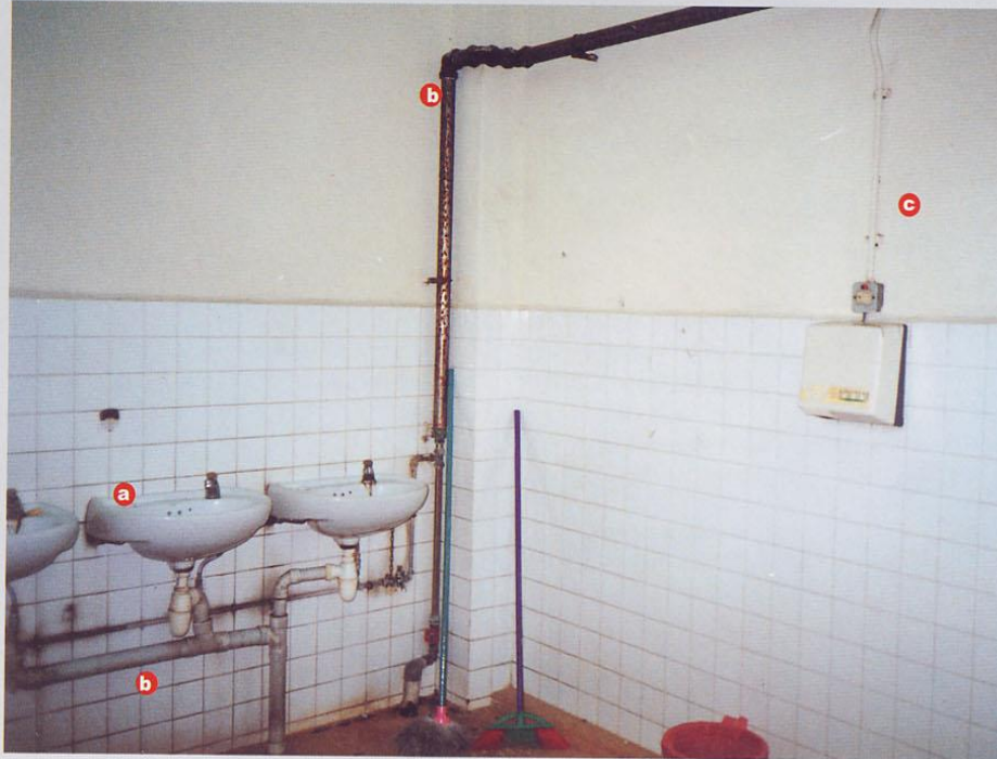
c. Surface Mounting of Cables
