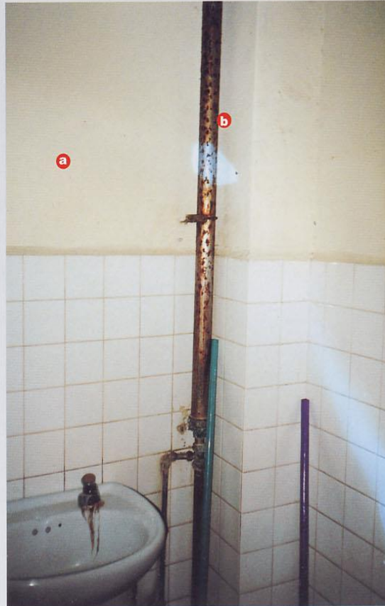
a. Painted Surface b. Exposed Piping
