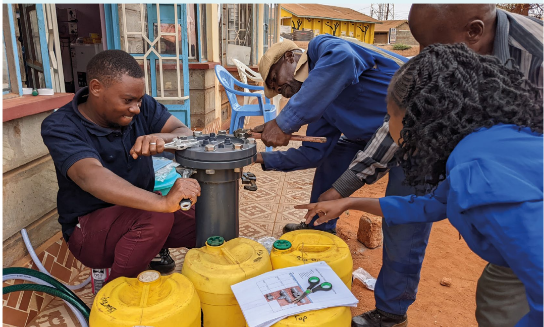
Photo shows members of a water service provider in April 2022 making pre-installation adjustments to a Venturi-style chlorinator developed by BlueTap.
