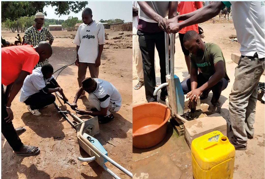
Photos show water service providers repairing handpumps.
