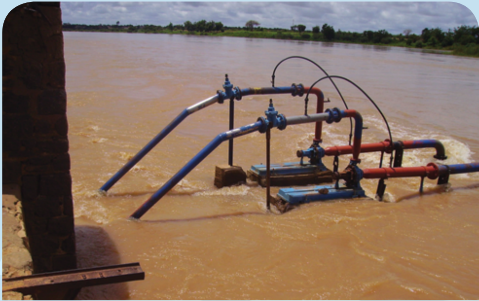
Flooded pumping equipment from Kayes water treatment station in Mali.
