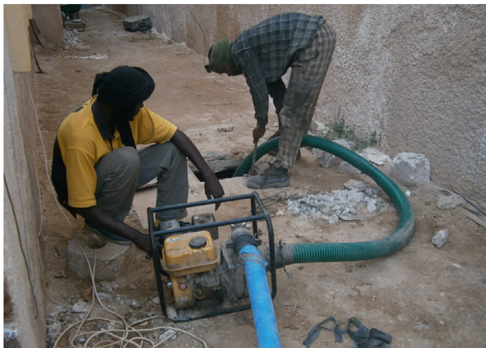
Manually emptying a septic tank in Mauritania
