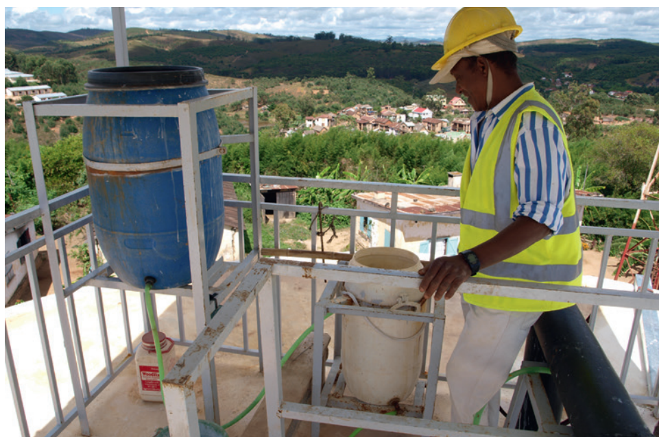
Chlorination of a drinking water storage tank in Madagascar
