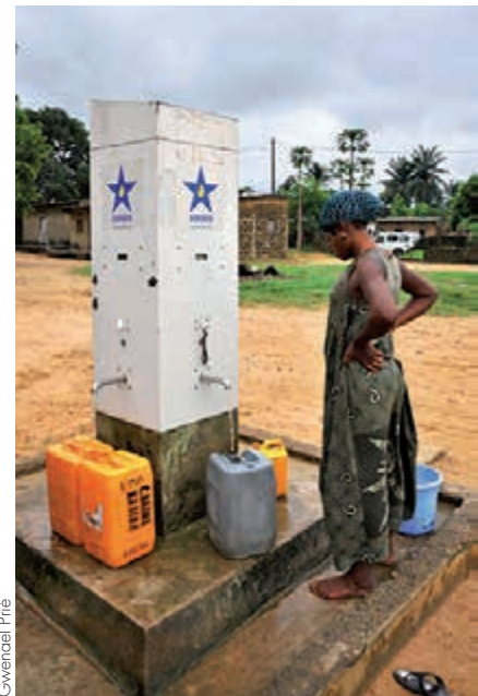
Sofoco public standpipe with prepaid magnetic card in DR Congo.
