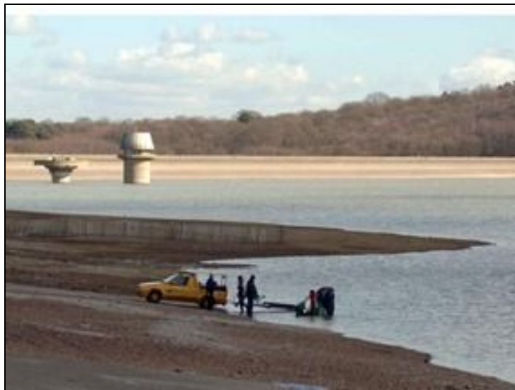
Figure 1.1 A depleted reservoir caused by drought conditions (Source: Halcrow Group)
