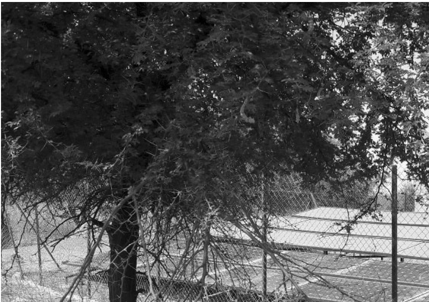
Figure 4.5 Shading of PV modules limiting power output
