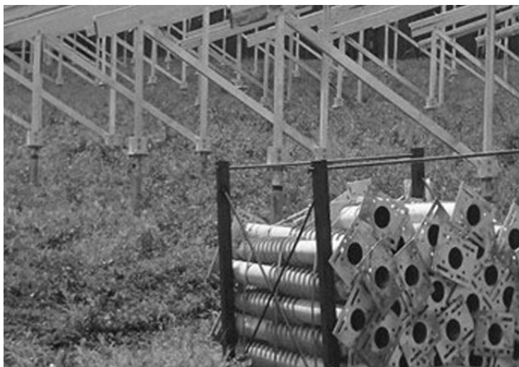
Figure 6.12 Example of ground screw structure
