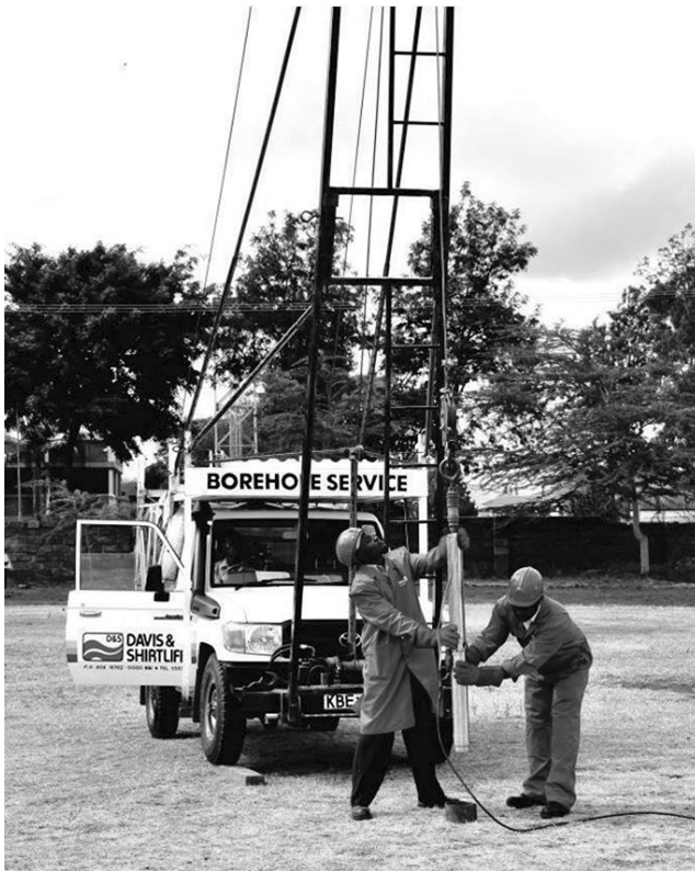
Figure 6.2 Pump installation using a hydraulic winch
