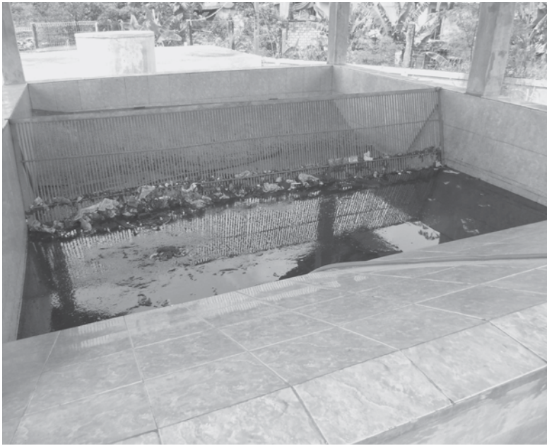
Photo 5.2 Vertical screen with no operator access
