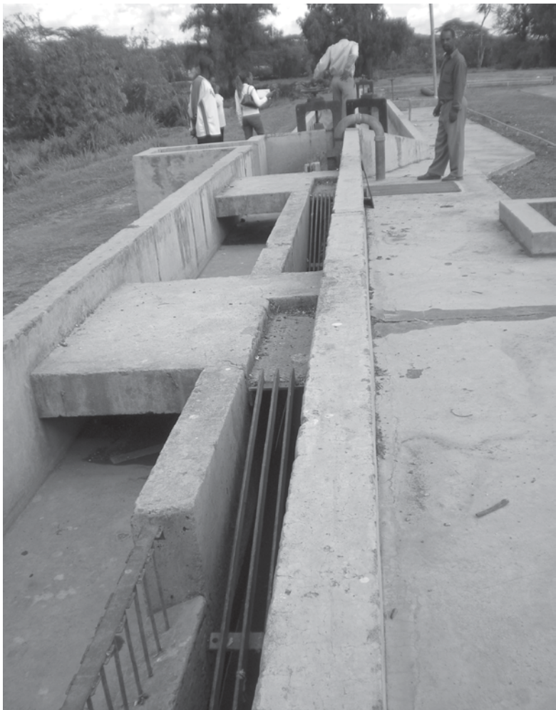
Photo 5.3 Inclined screen with operator access
