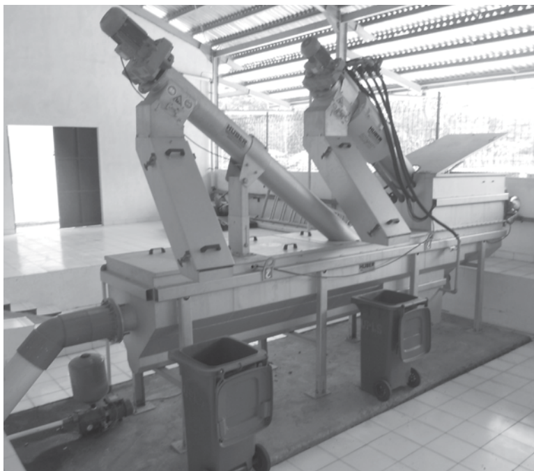
Photo 6.8 Combined mechanical screening and grit removal, Jakarta
